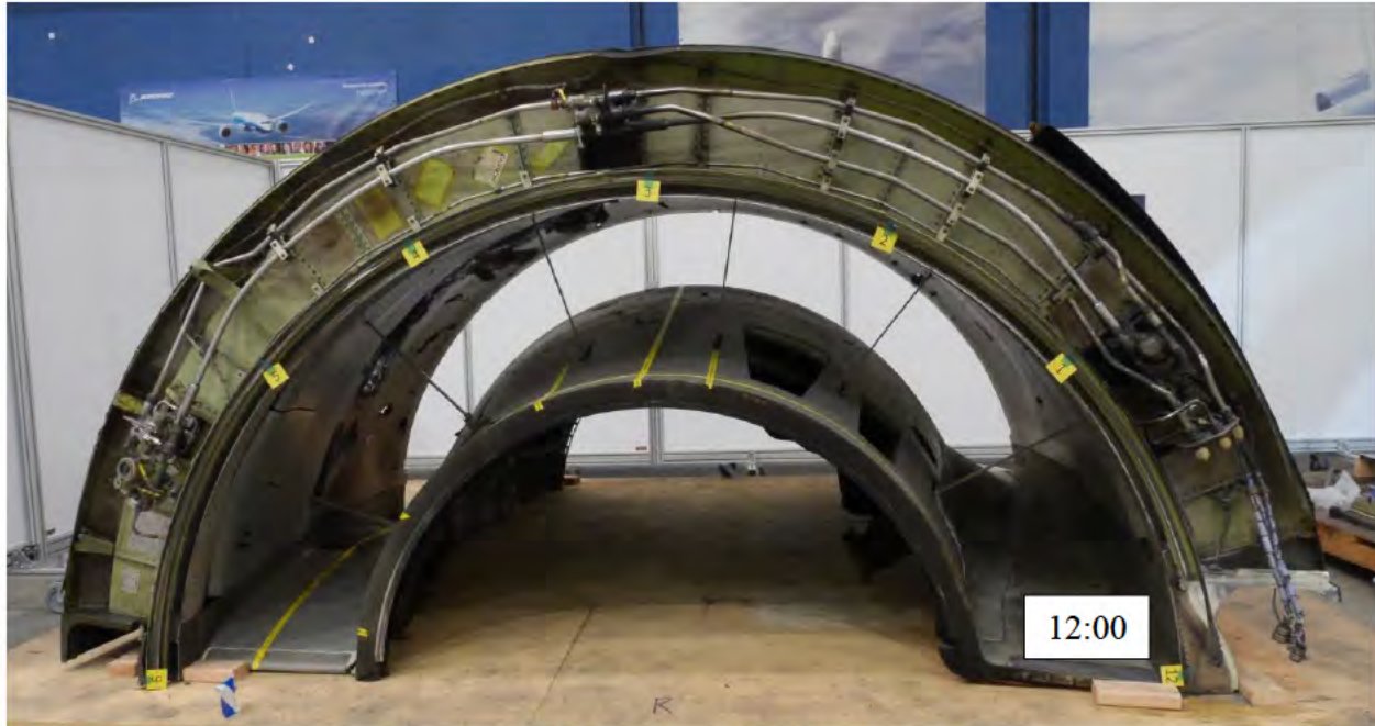
Figure 1. Right Thrust Reverser (P/N 315W3001-4AA SN 000002). A short fracture runs from the edge of the part at the 12:00 clock position, extending for approximately 1.7 inches.
