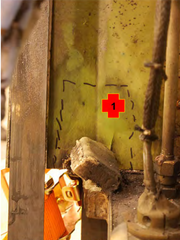
Figure 83: Outboard (right) thrust reverser crack at 12:00.
