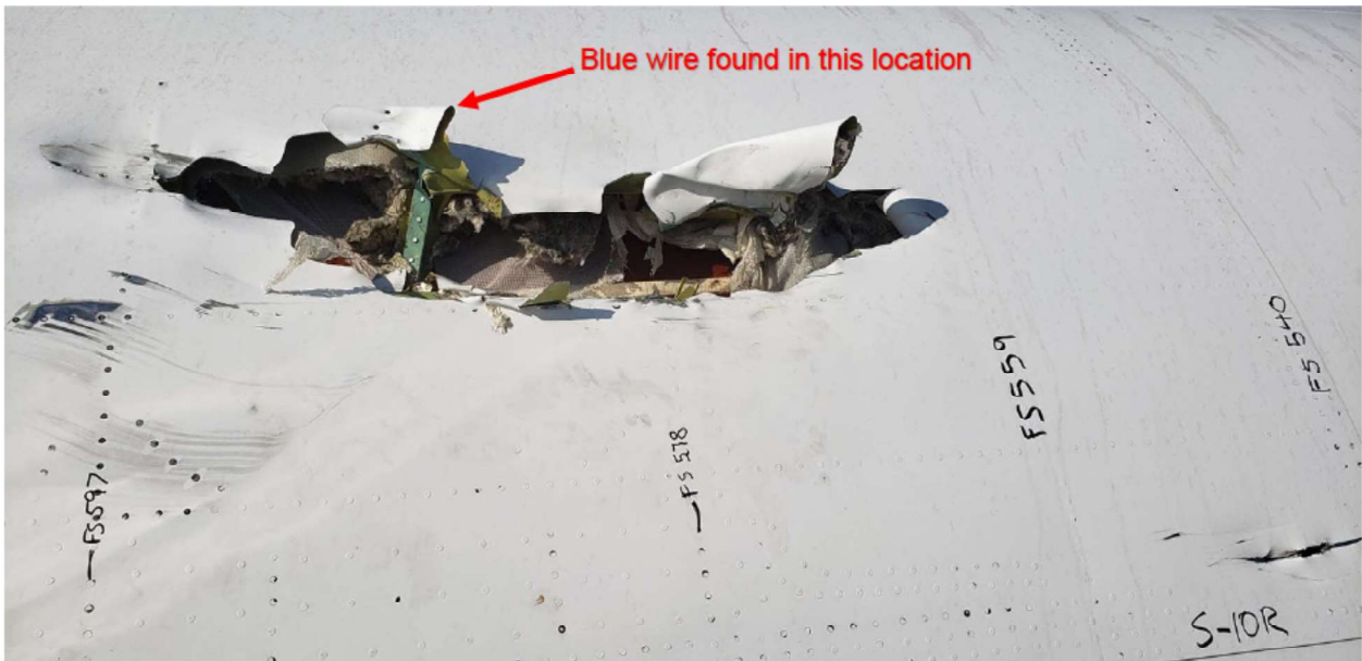
Figure 2 – Image of damage area provided by Boeing ASI
