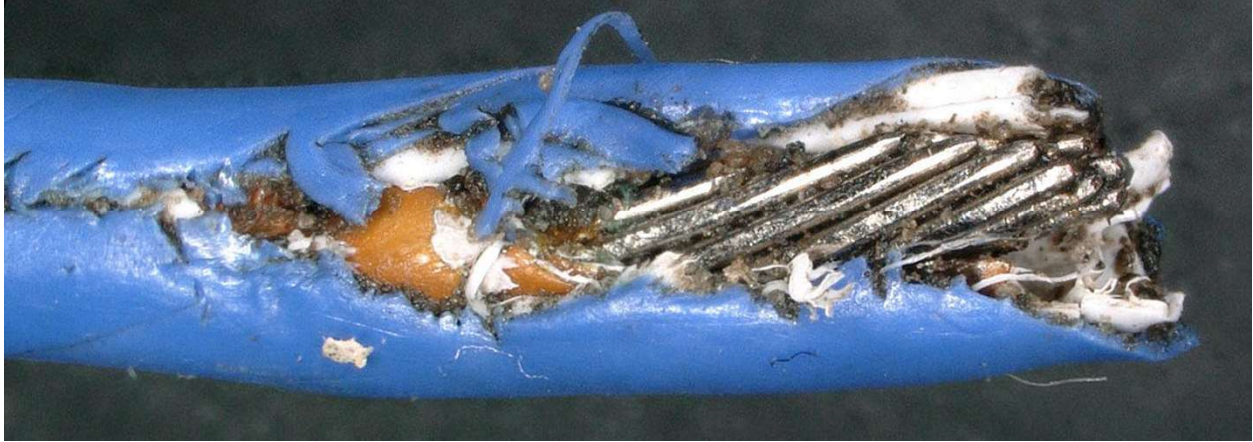
Figure 15 – RMLG blue wire fractured end
