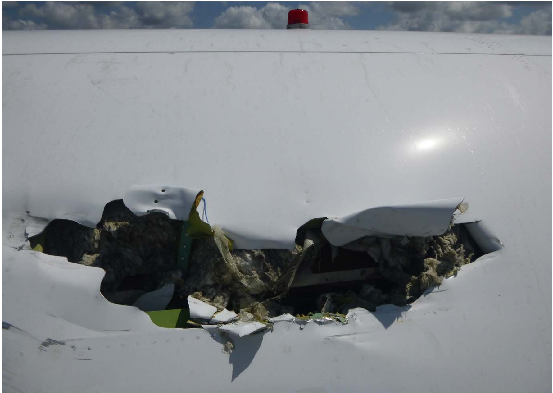
Figure 7 – Hole in fuselage above right forward overwing emergency exit
