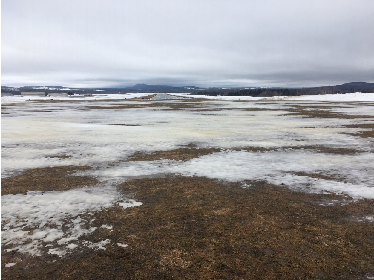
Photo 8. Snow cleared between the localizer antenna and runway (courtesy PQI).
