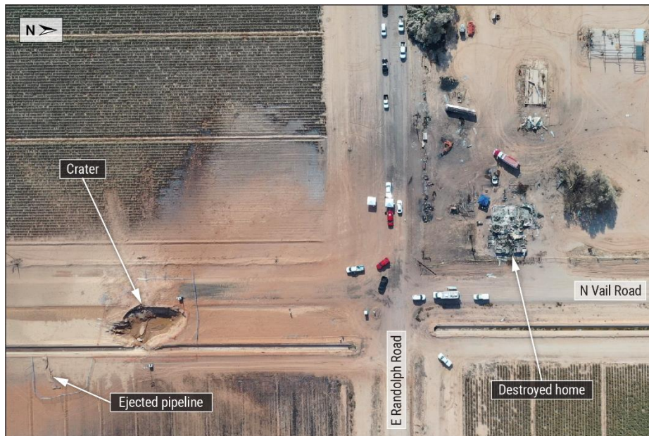
Figure. Aerial image of accident scene following the explosion. (Courtesy of the Pinal County Fire Investigation Task Force)
