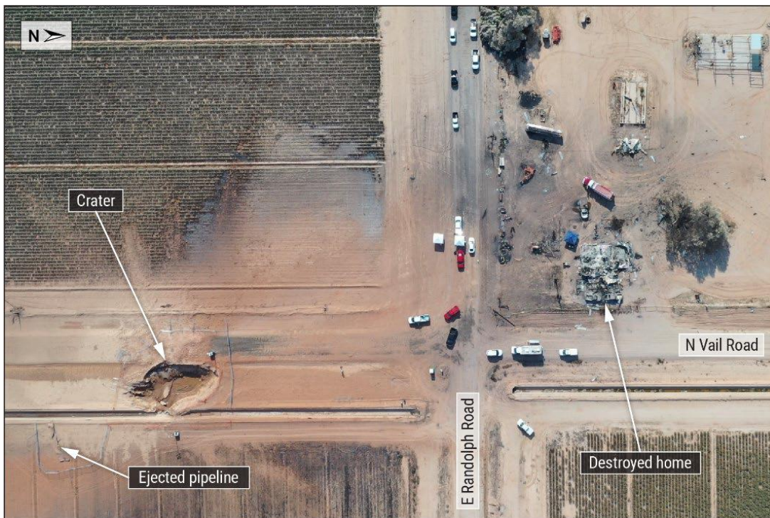
Figure 1. Aerial image of accident scene following the explosion. (Courtesy of the Pinal County Fire Investigation Task Force)
