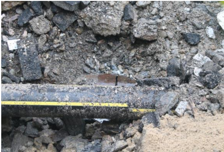
Figure 9: The exposed 8-inch HDPE gas main and 12-inch cast iron water main cracked location. Source: NYPSC
