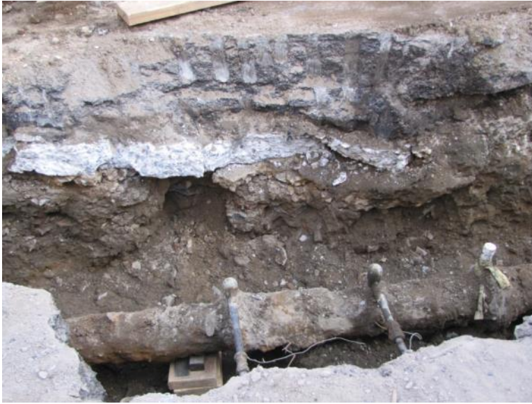
Figure 28: Service tees to 1646 and 1644 Park Avenue below about 12 inches of concrete road underlay with about 18 inches thick asphalt paving.
