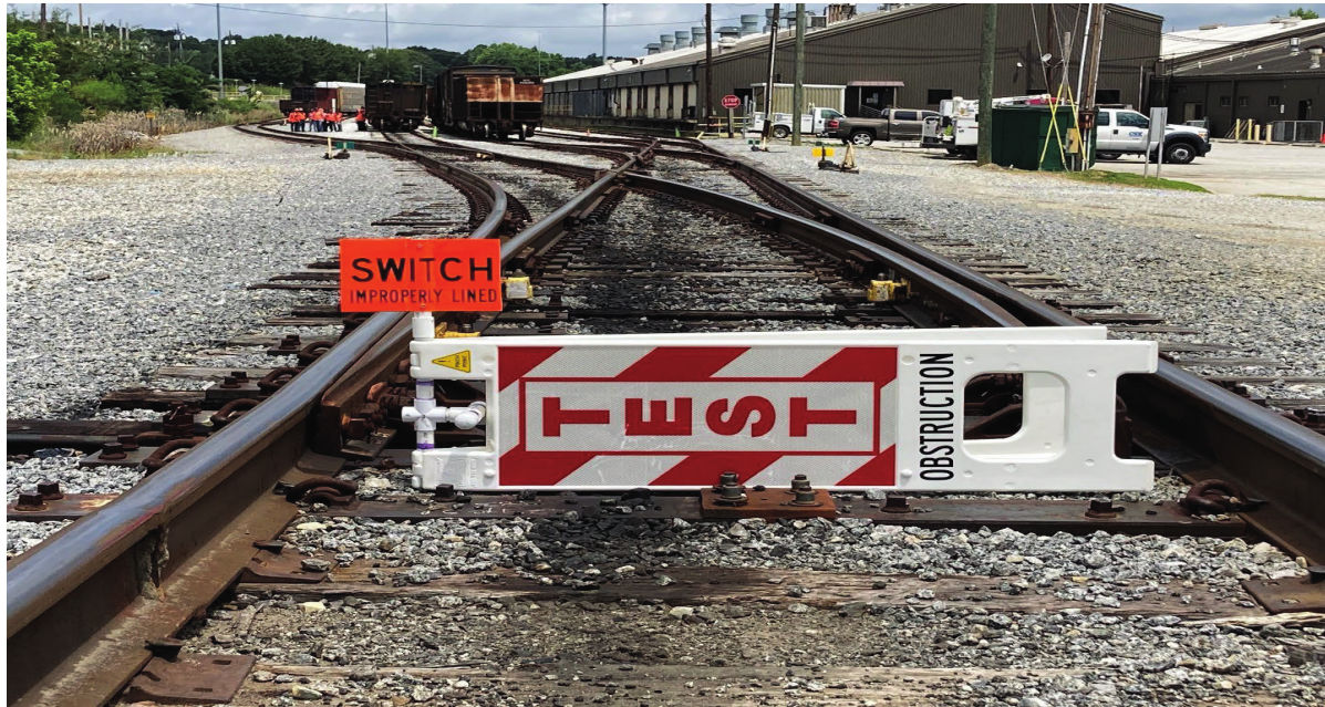
Example of simulated improperly lined switch.
