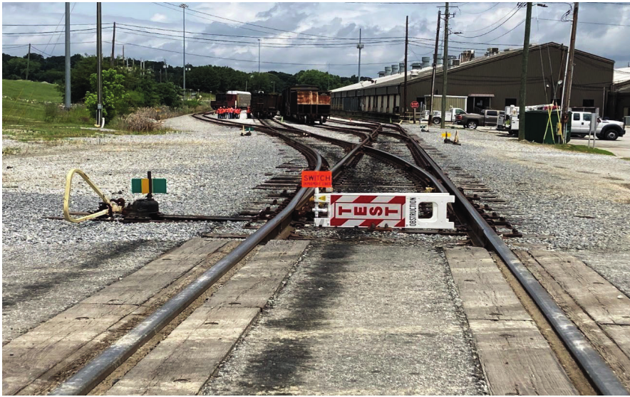
Example of simulated improperly lined switch.
