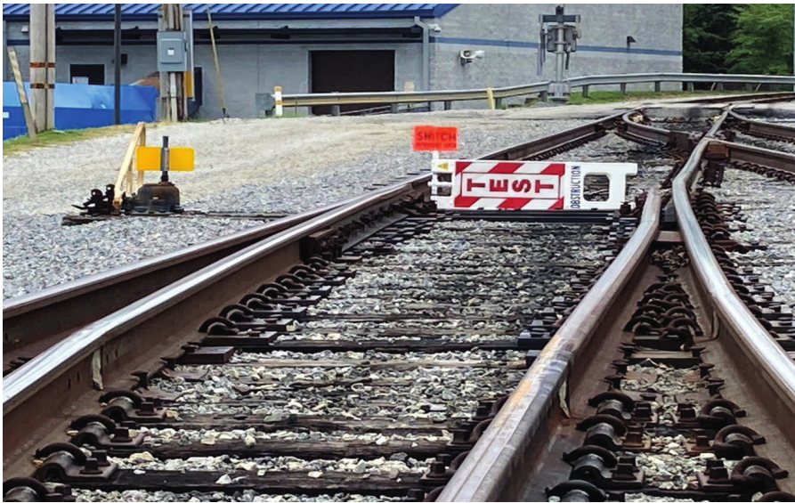
Example of simulated improperly lined switch.
