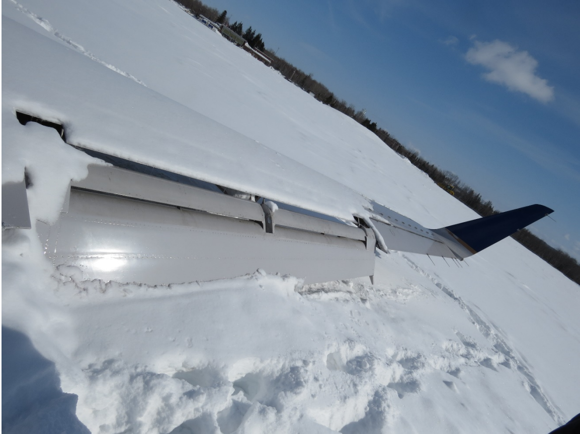
Figure 9 Right wing outboard flap and aileron
