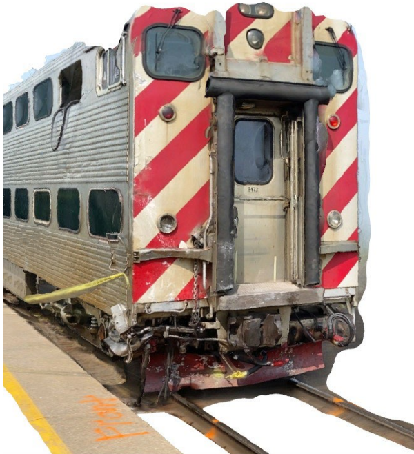
Figure 3. Screen capture of 3D point cloud depicting damage incurred during the collision.
