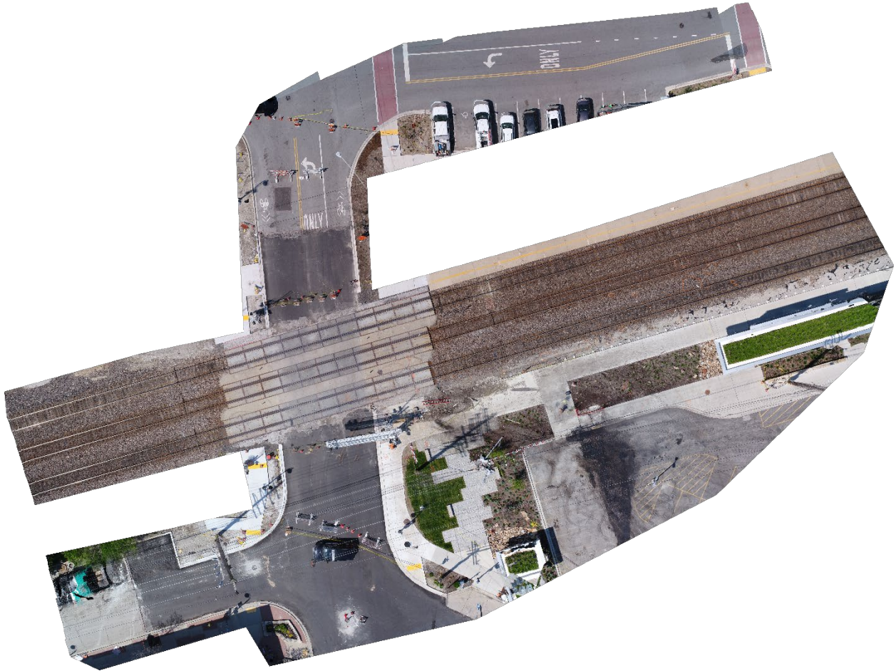
Figure 10. Orthomosaic image depicting the overhead view of the grade crossing.
