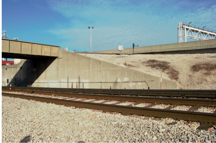
Figure 4 Photograph looking from the accident scene showing the yellow line tracks and the path taken by the emergency responders to access the scene and used by the responders to evacuate the injured. (Source: NTSB)
