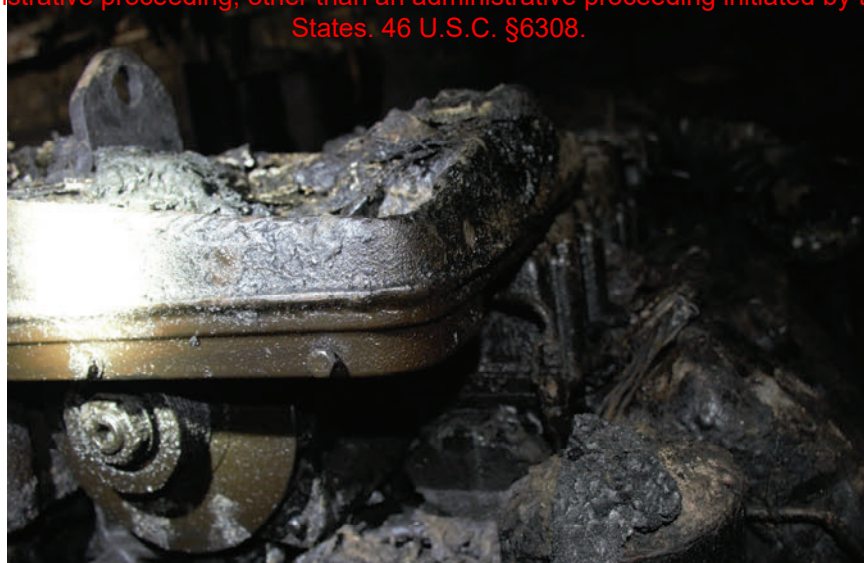
Damage to the Top of the Port Side Engine
