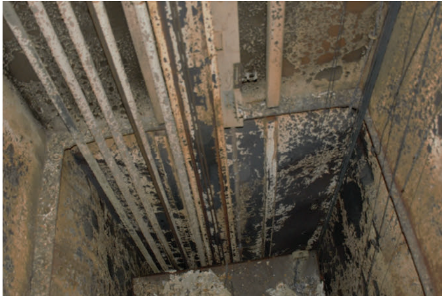
Inside of the Elevator Shaft
