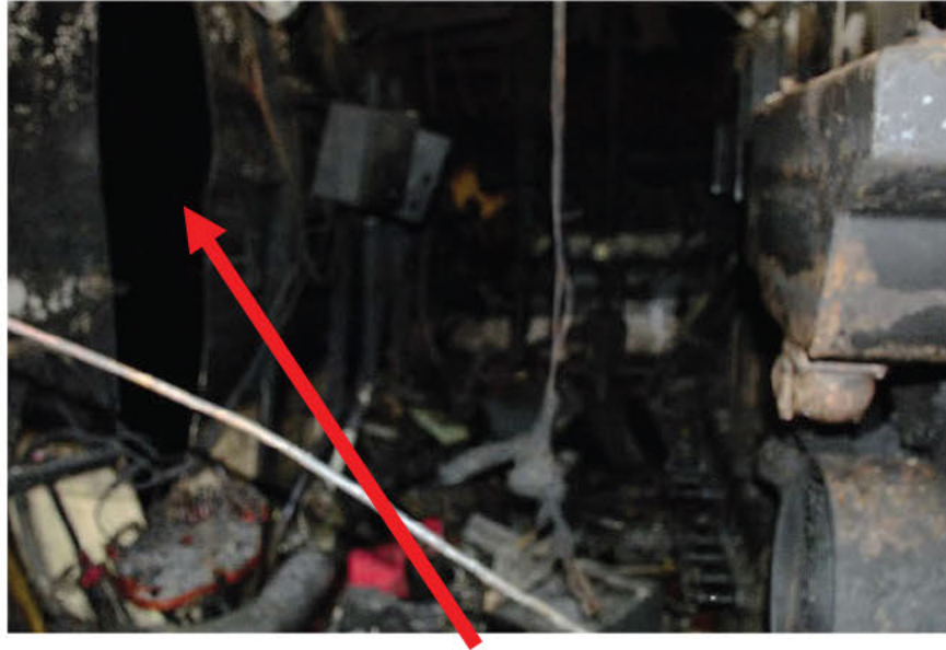
Opening in Starboard Tank
