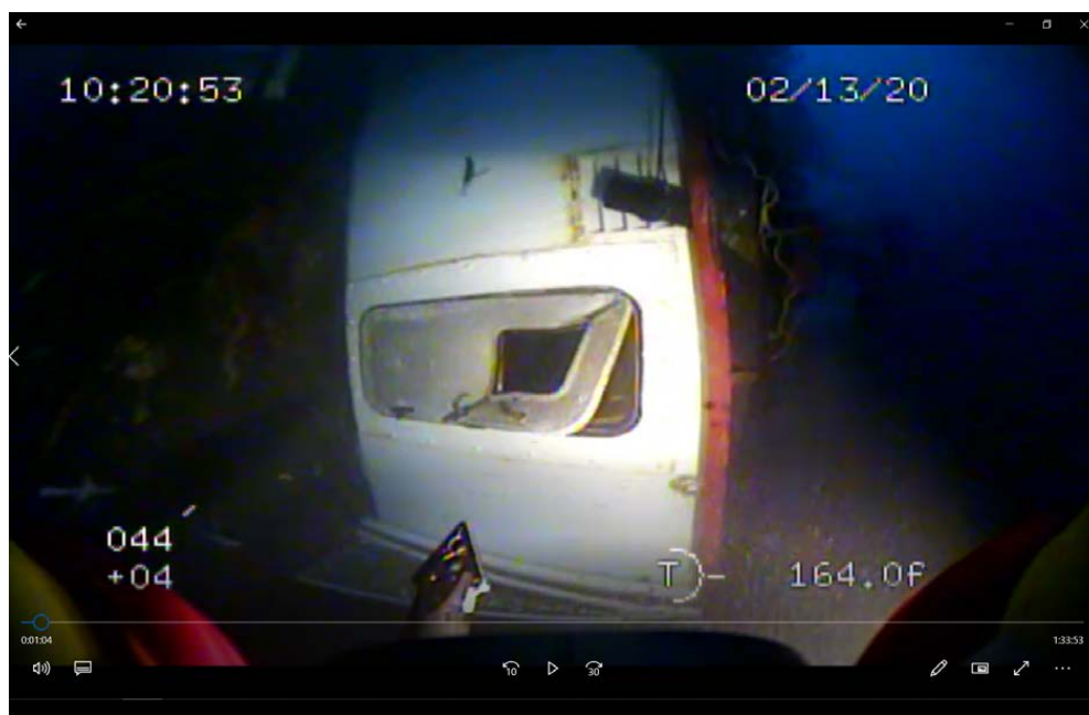
Figure 9: A man door located at the starboard stern of the accommodation suffered damage.
