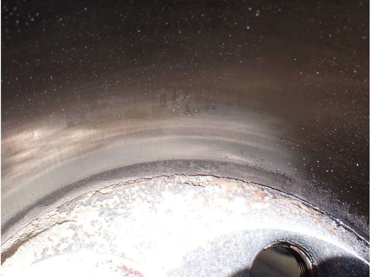
Figure 4: Corrosion of the #1 cylinder head and a crack between the cylinder head and bore.
