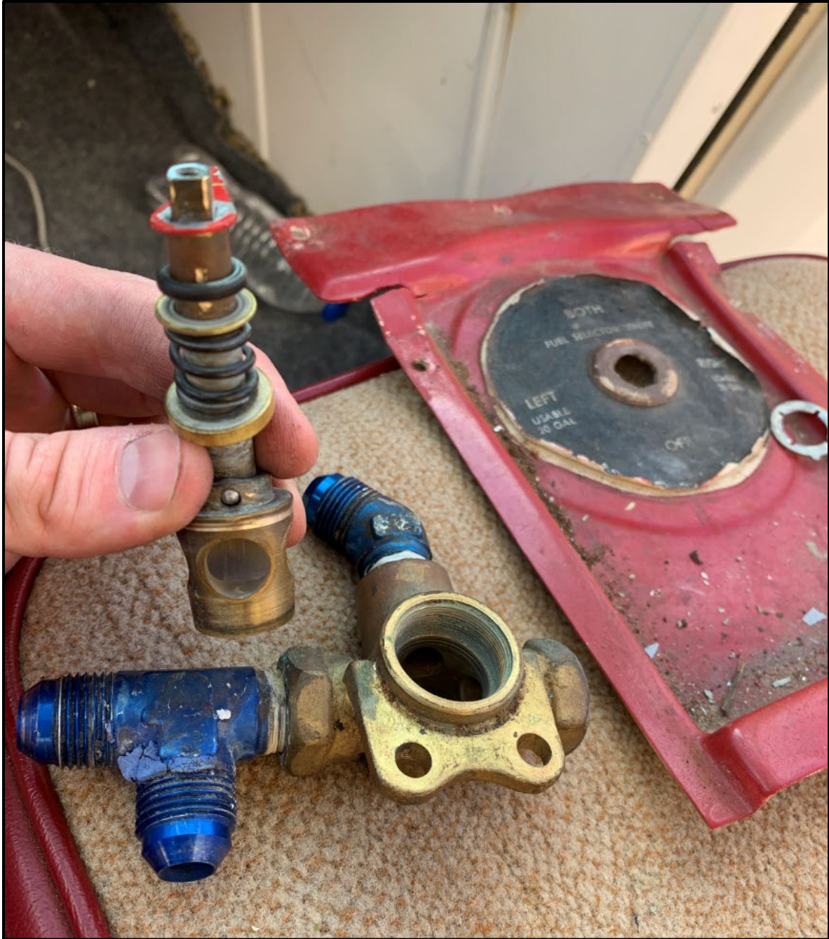
Figure 2 – View of the removed fuel selector.
