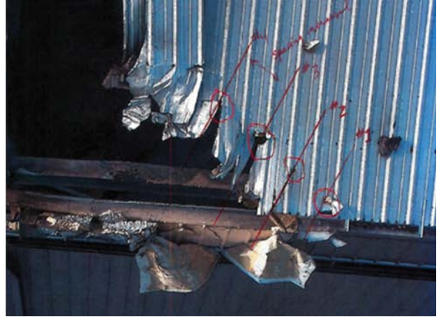
Figure 4. Propeller blade strikes at entry hole
