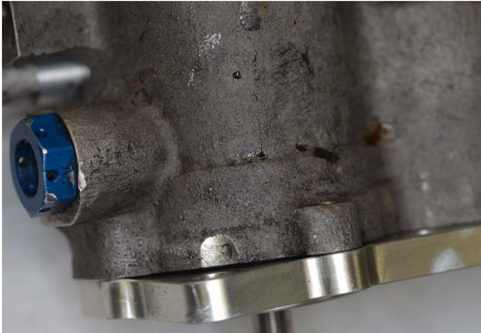
Figure 64. Deformed baseplate, FCU S/N 20565991
