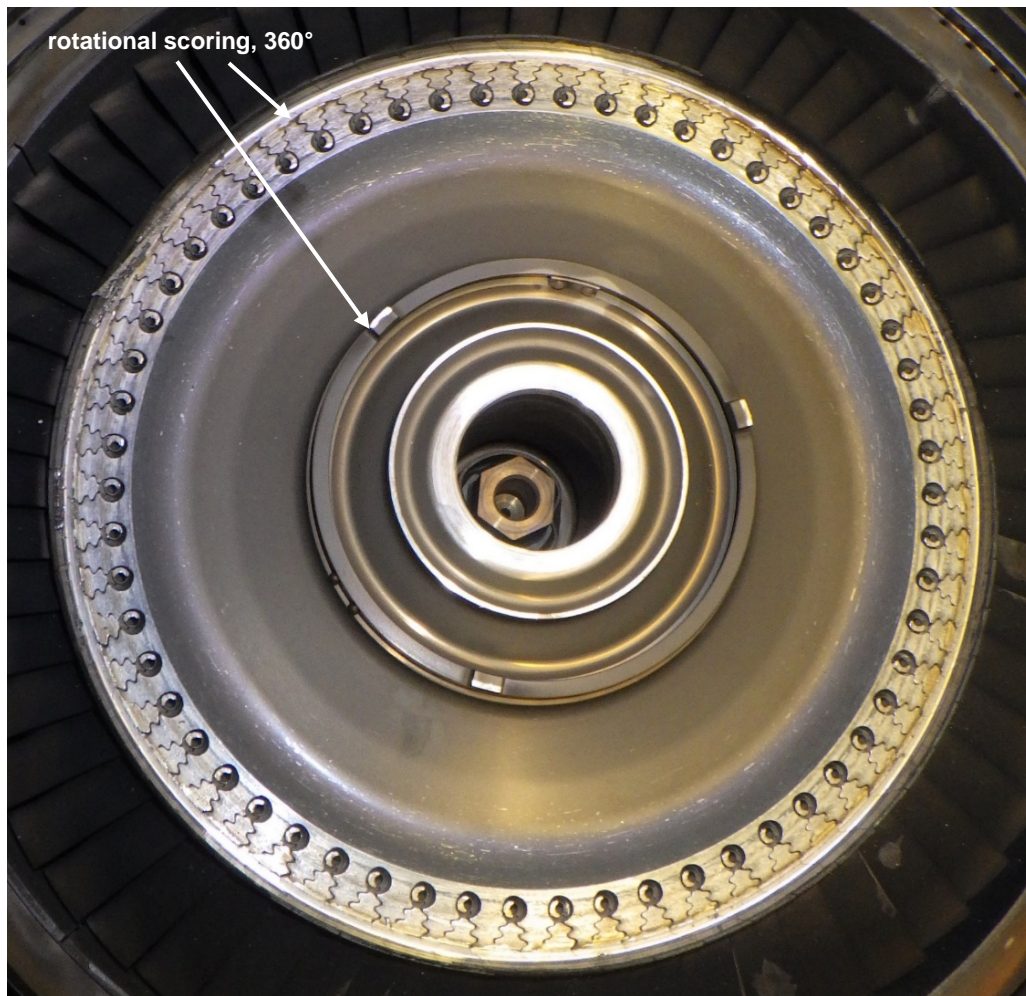
Figure 37. Downstream face of CT showing 360° scoring in the fir tree root area and tooling lugs
