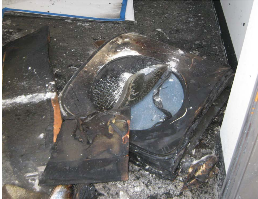
Figure 20 - Emergency Exit Hatch
