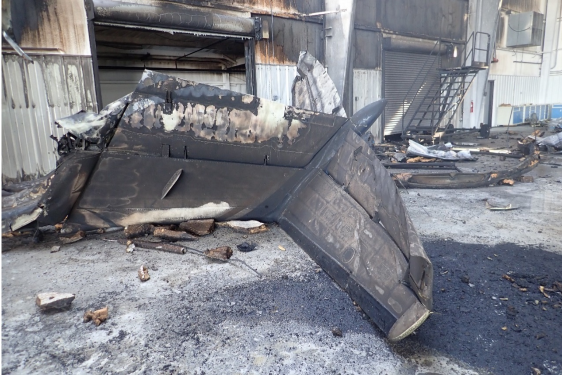
Figure 12 - Vertical Stabilizer and underside of horizontal stabilizer, in hangar.
