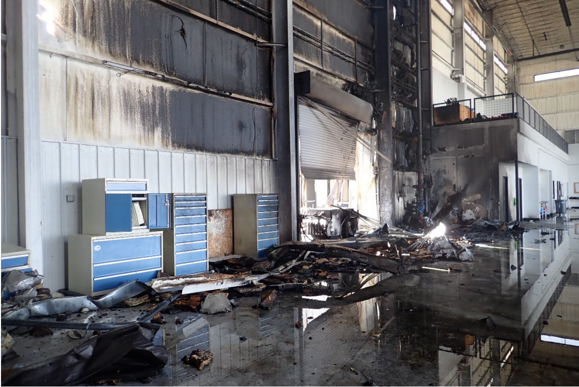
Figure 8 - Inside the hangar, looking at the roll-up door.
