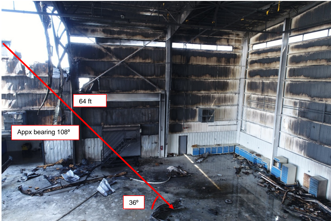
Figure 8 – Angle from approximate center of impact to first significant gouge
