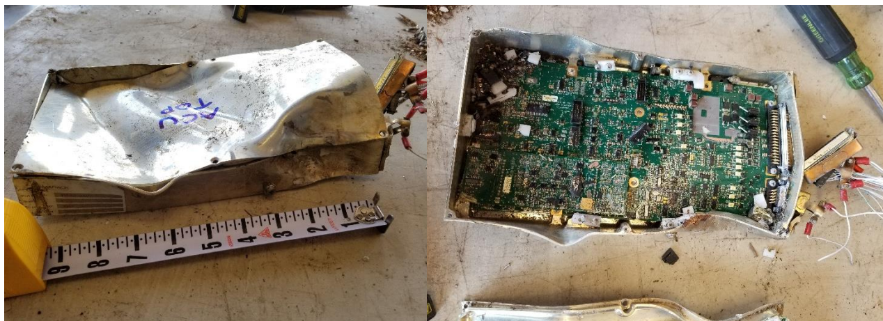
Figure 2-1 ACU as-found condition (external view left, internal view right)
