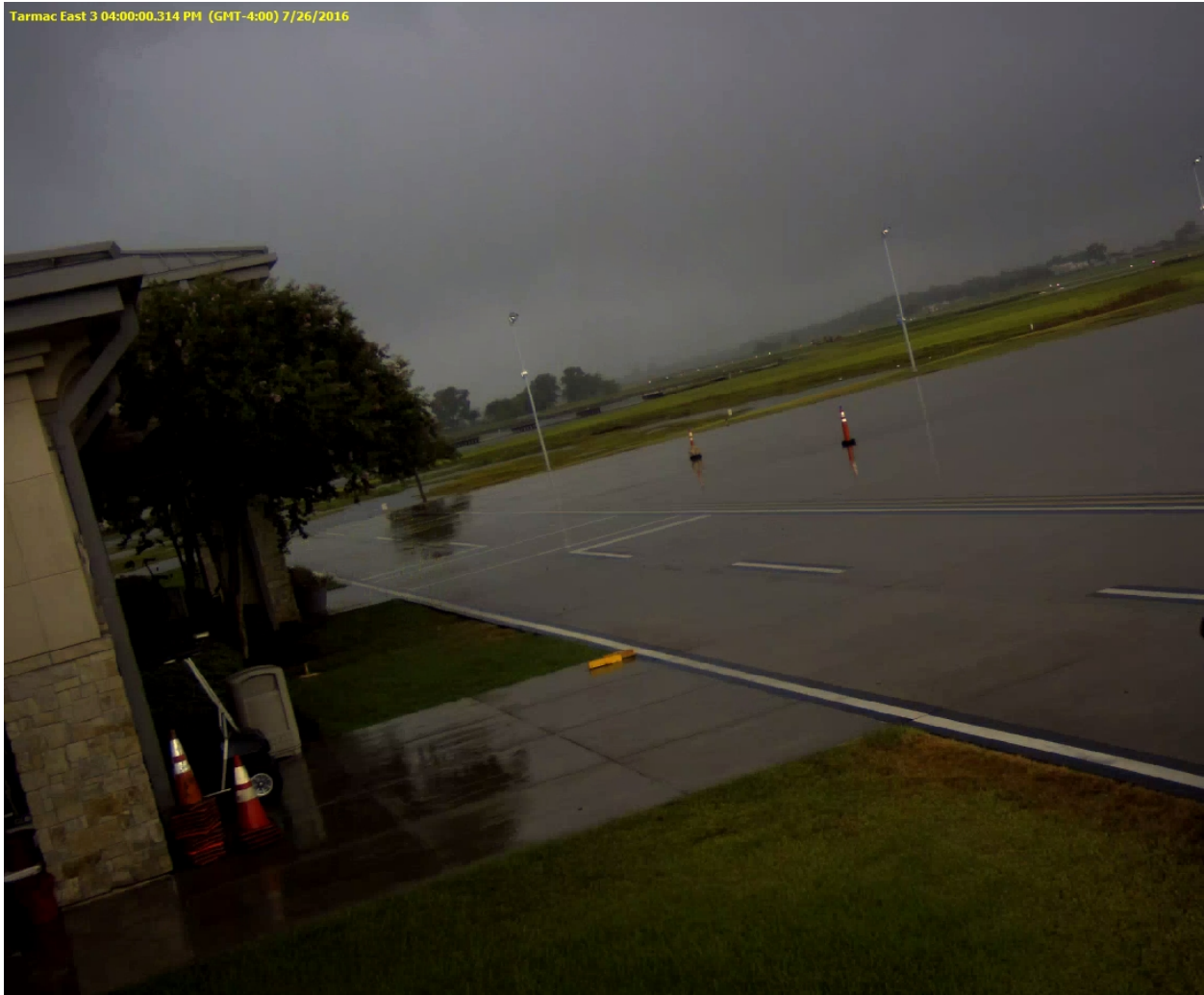
Figure 45 – SGR Security Camera image looking south-southwest towards the south end of the SGR runway at 1500:00 CDT
