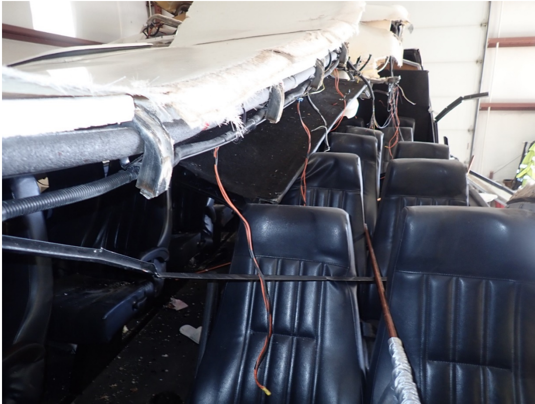
Figure 5: View of the damage and integrity loss to the roof structure of the Freightliner
