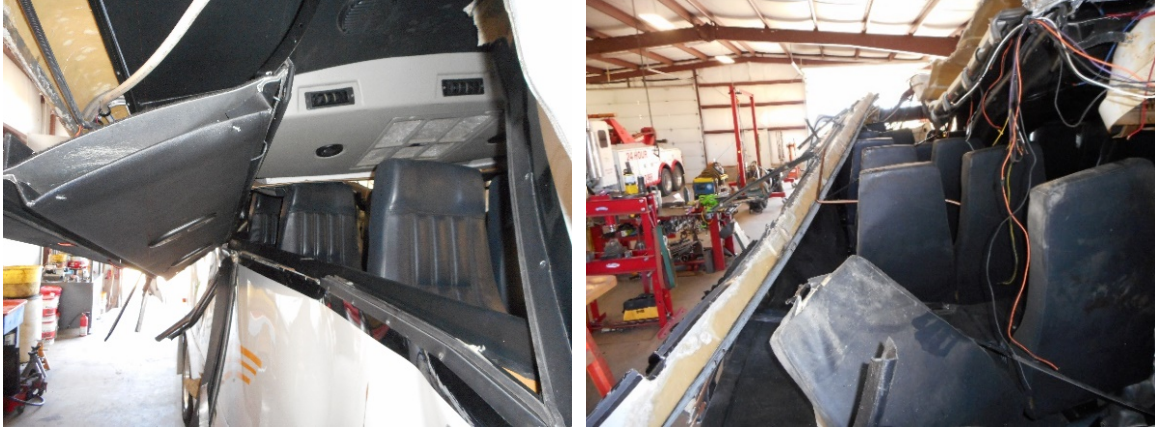
Figure 3. View looking aft at lateral roof shift on right side. Figure 4. View of lateral roof shift on left side.
