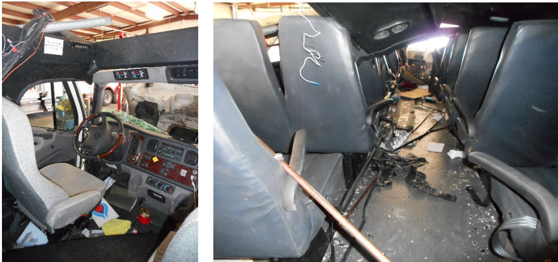
Figure 5. Interior view of missing roof above driver seating. Figure 6. View looking forward of roof collapse.
