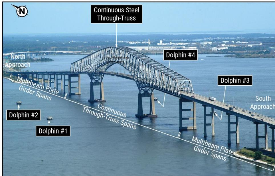
**Figure 2.** Key Bridge (source: MDTA revised).
