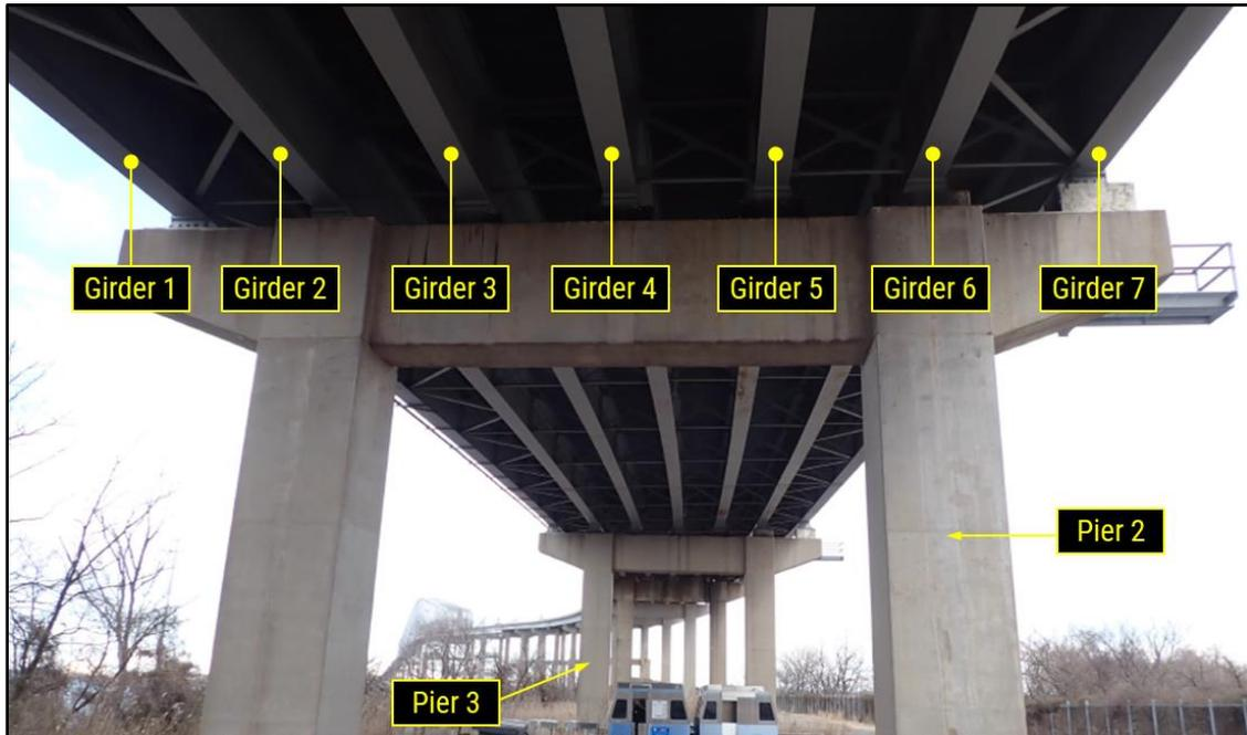
**Figure 5.** Continuous painted steel girders (source: MDTA).
