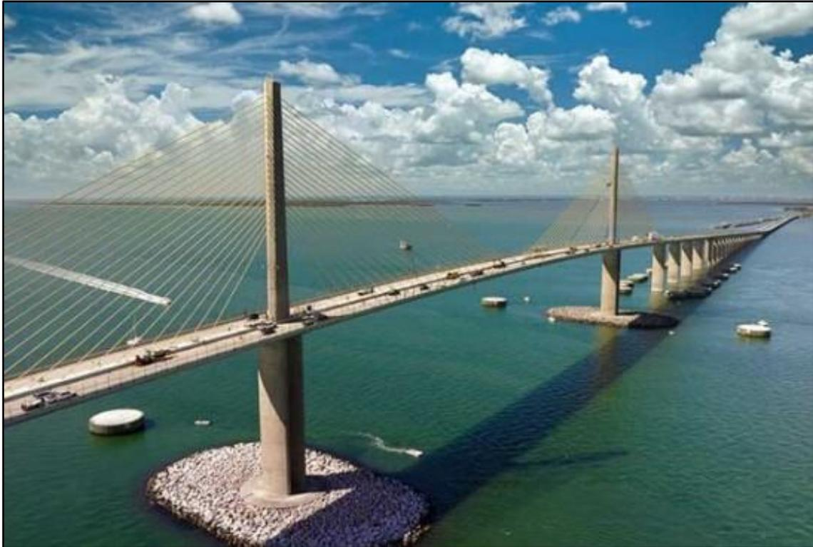
**Figure 65:** Aerial view of the new pier protection system for the Sunshine Skyway Bridge in Tampa Bay, FL, after the collapse (source: FDOT).
