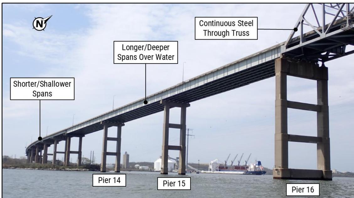
**Figure 6.** Three types of spans at the Key Bridge (source: MDTA).
