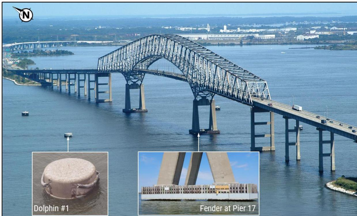
**Figure 7.** Pier 17 protection from outbound vessels transiting the Key Bridge (source: MDTA revised).
