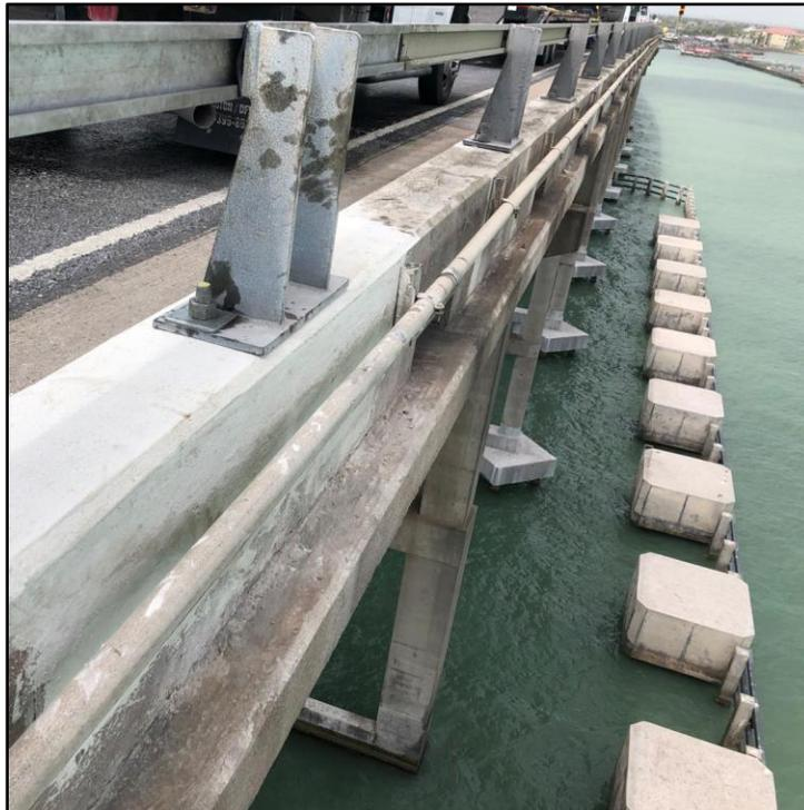
**Figure 72:** New pier protection system for the Queen Isabella Causeway (source: TxDOT).
