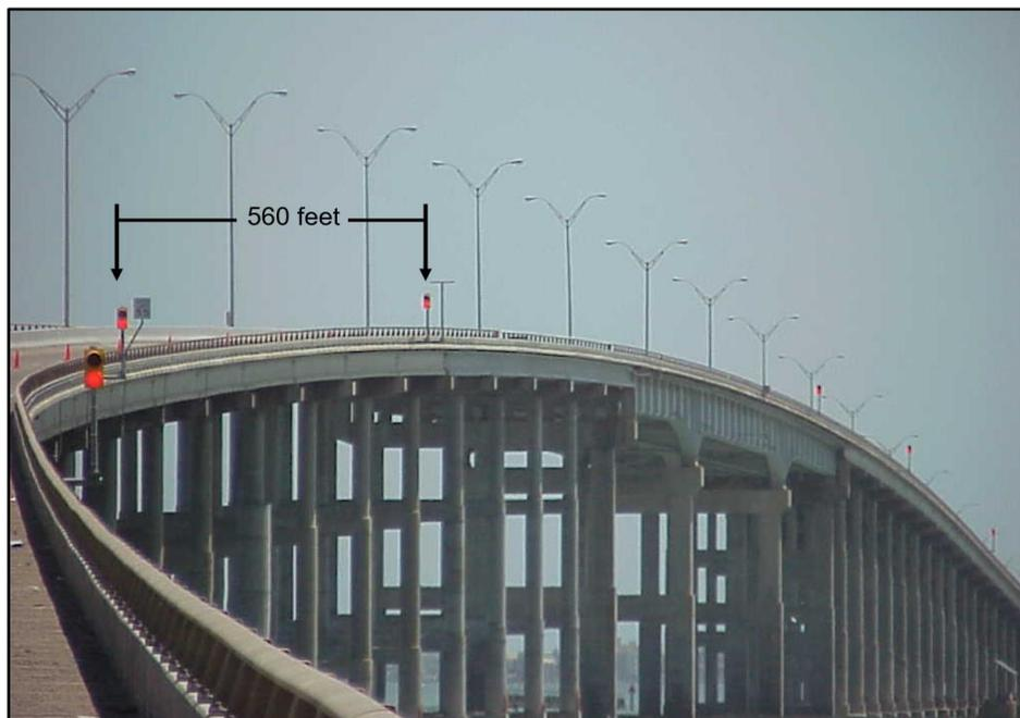
**Figure 68:** Early warning collapse detection system on the Queen Isabella Causeway bridge (source: TxDOT).
