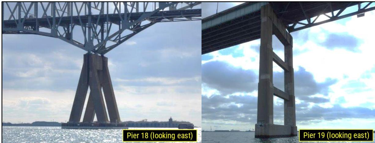
**Figure 4.** Rigid frame reinforced concrete pier (left) and two-column pier (right) (source: MDTA)
