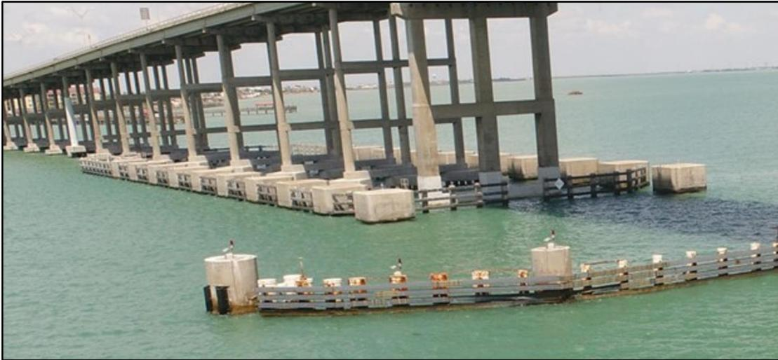
**Figure 71:** New pier protection system for the Queen Isabella Causeway (source: TxDOT).
