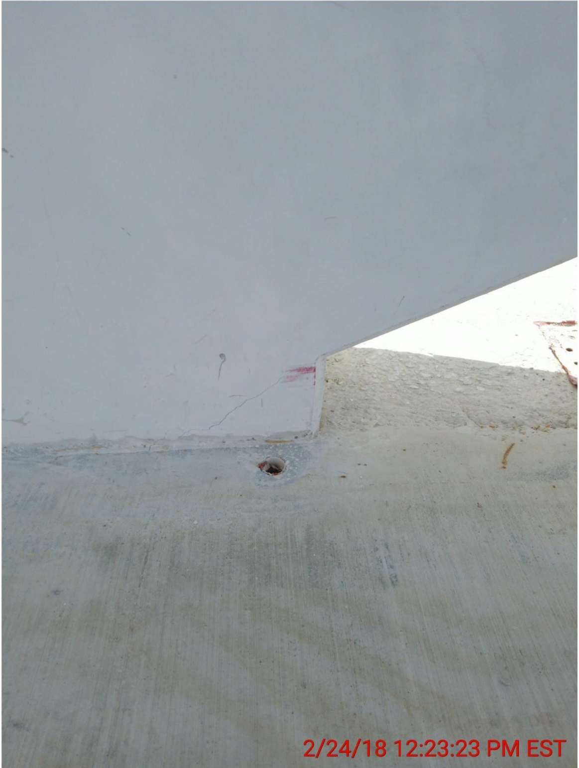
Bridge Factors Photo 36 – View of crack at the bottom of diagonal support #2 on north side looking to the south in casting yard on 2/24/18 at 12:23:23 p.m. (Source: Munilla Construction Management, MCM)
