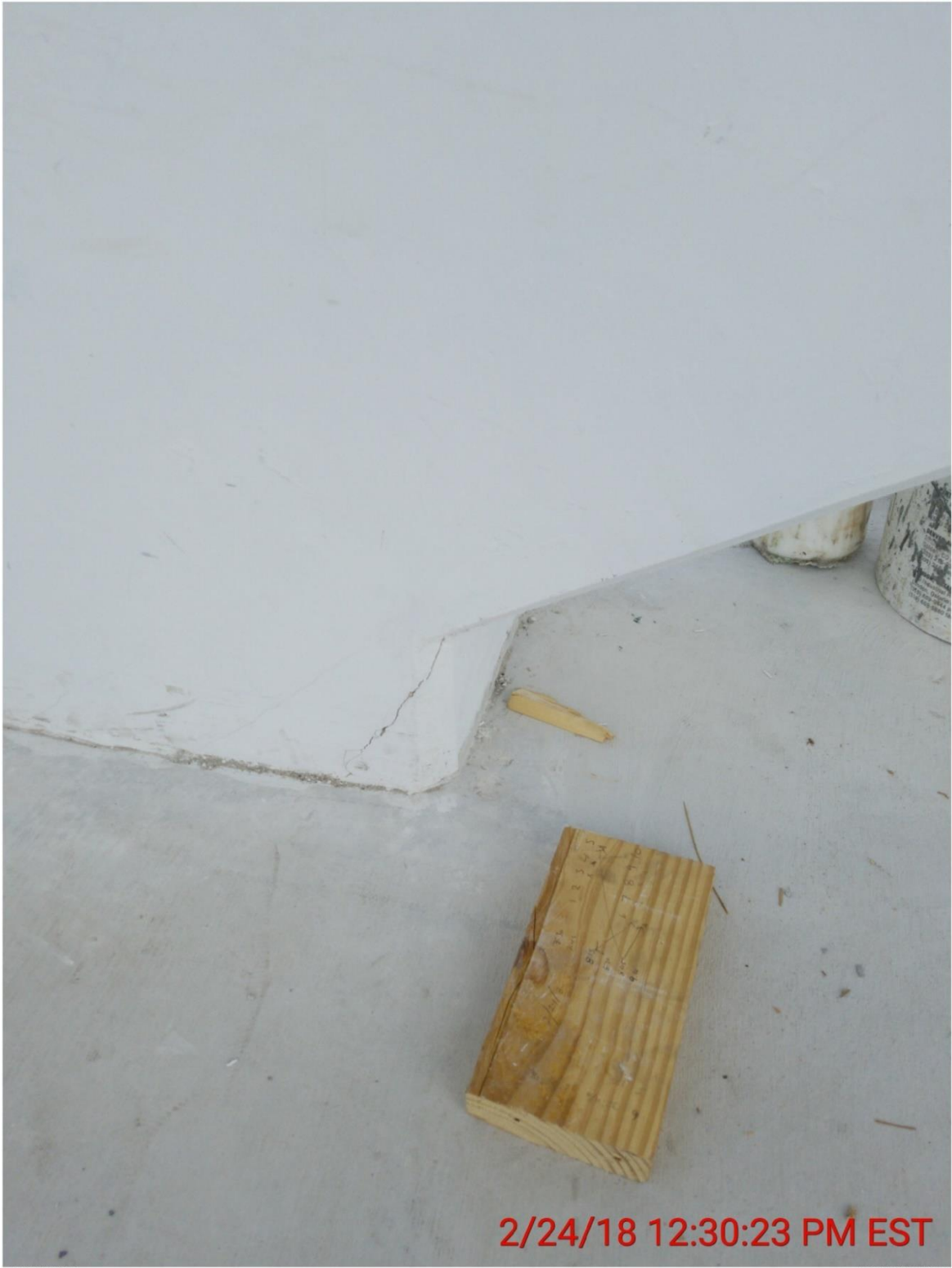
Bridge Factors Photo 39 – View of crack at the bottom of diagonal support #11 on south side looking to the north in casting yard on 2/24/18 at 12:30:23 p.m. (Source: Munilla Construction Management, MCM)
