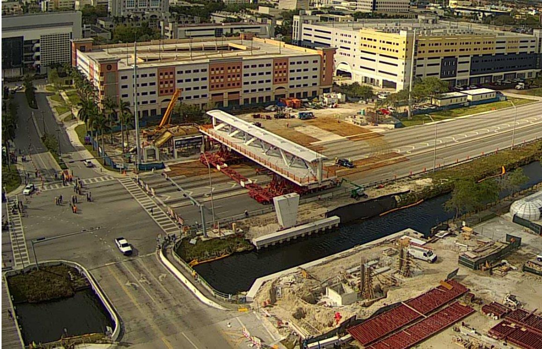
Bridge Factors Photo 108 – View of transporters moving the pedestrian bridge into place on the bridge piers looking to the southwest (Source: FIU)
