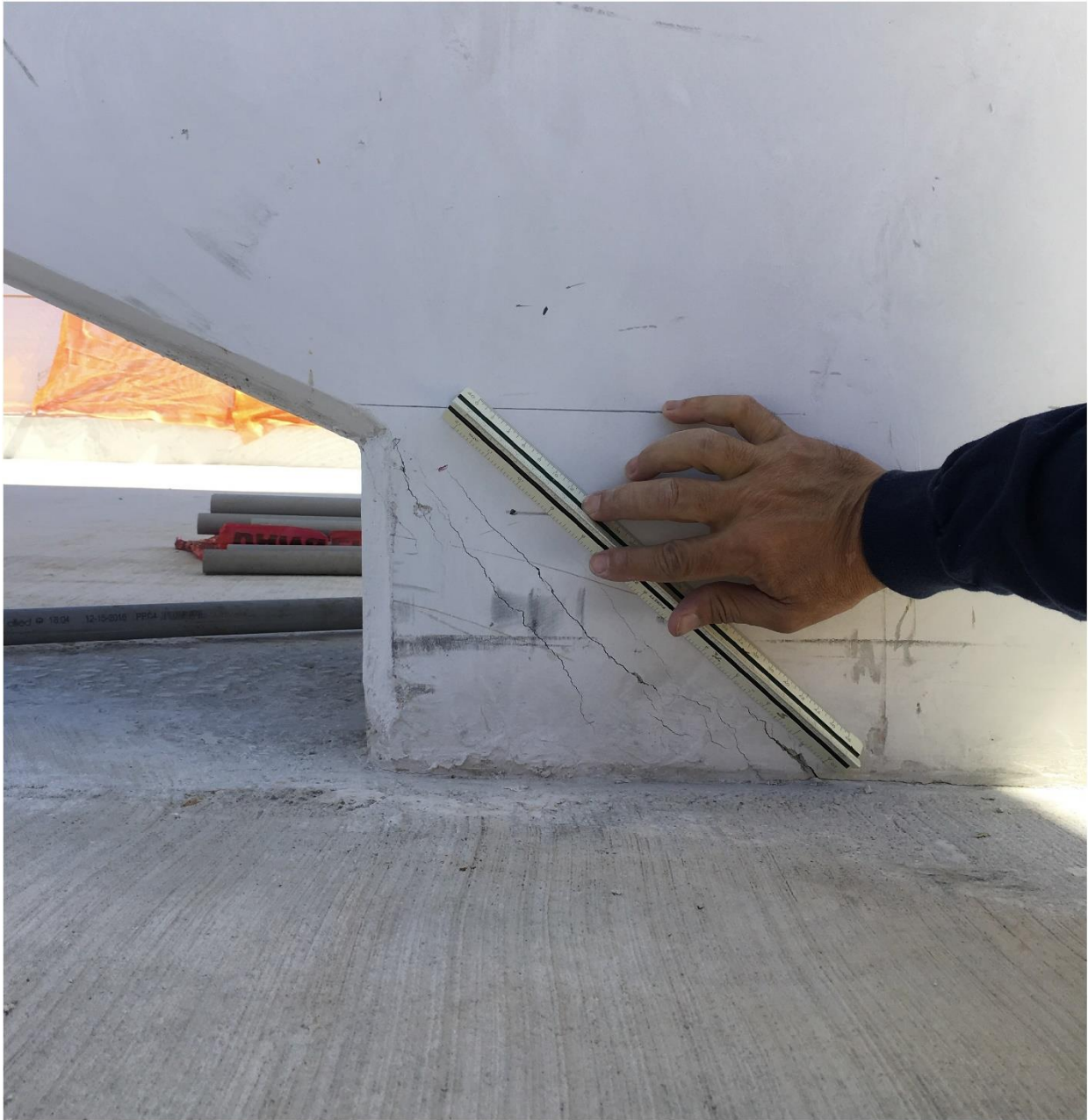
Bridge Factors Photo 86 – View of cracks at the bottom of diagonal support #2 on west side looking to the east on 3/13/18 at 1:44:53 p.m. (Source: Munilla Construction Management, MCM)
