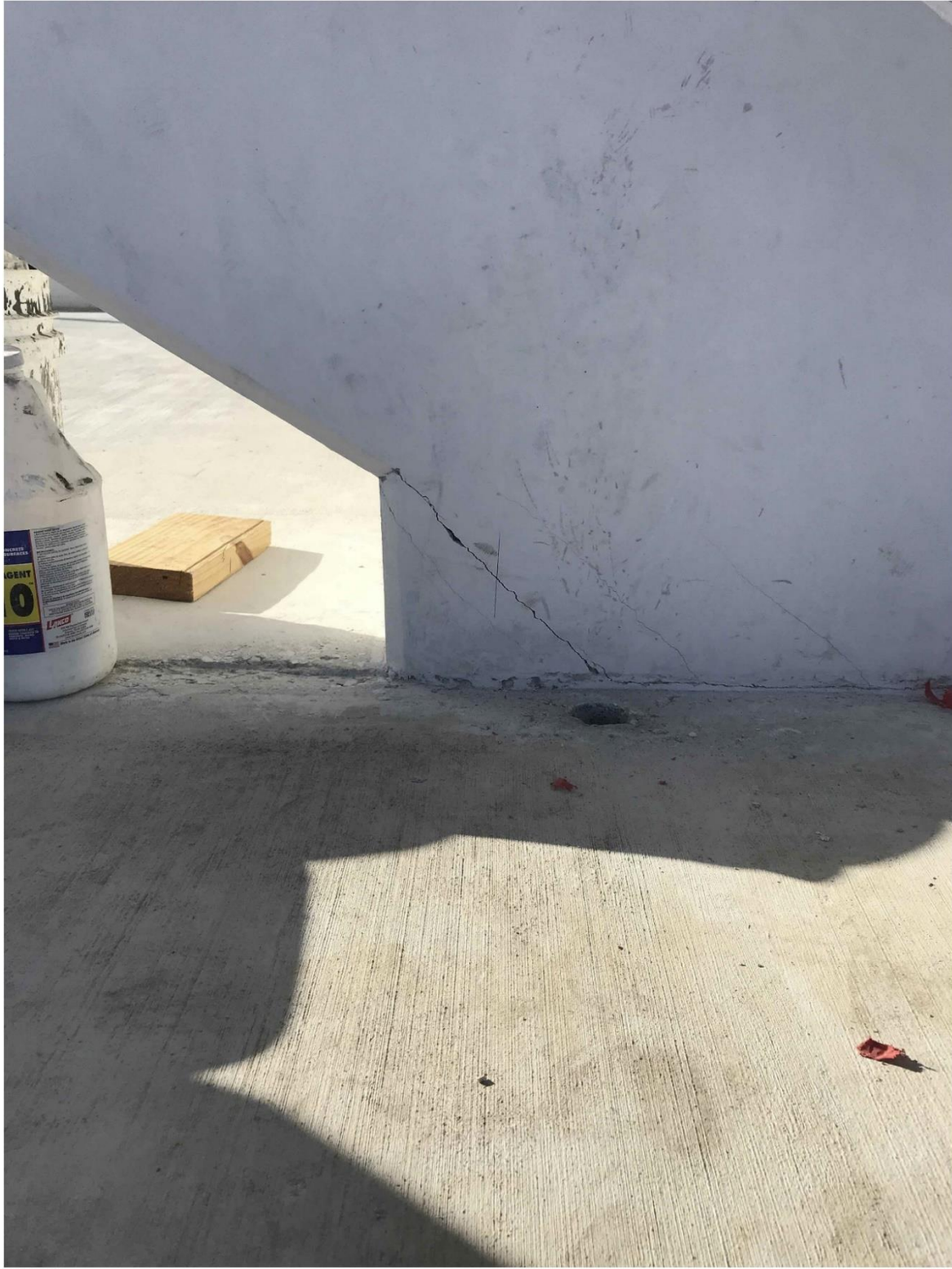
Bridge Factors Photo 42 – View of crack at the bottom of diagonal support #11 on north side looking to the south in casting yard on 2/26/18 at 8:38:16 a.m. (Source: Munilla Construction Management, MCM)
