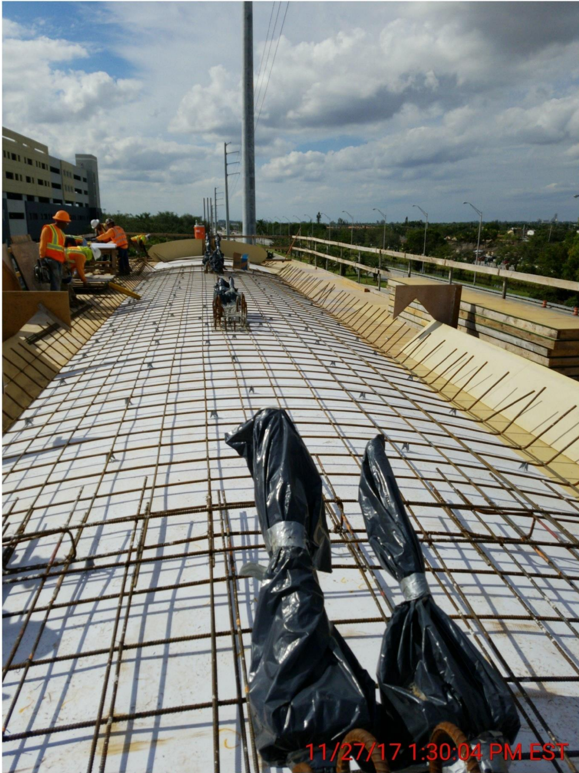
Bridge Factors Photo 22 – View of reinforcement bars being set on top of canopy on 11/27/17 at 1:30:04 p.m. (Source: Munilla Construction Management, MCM)
