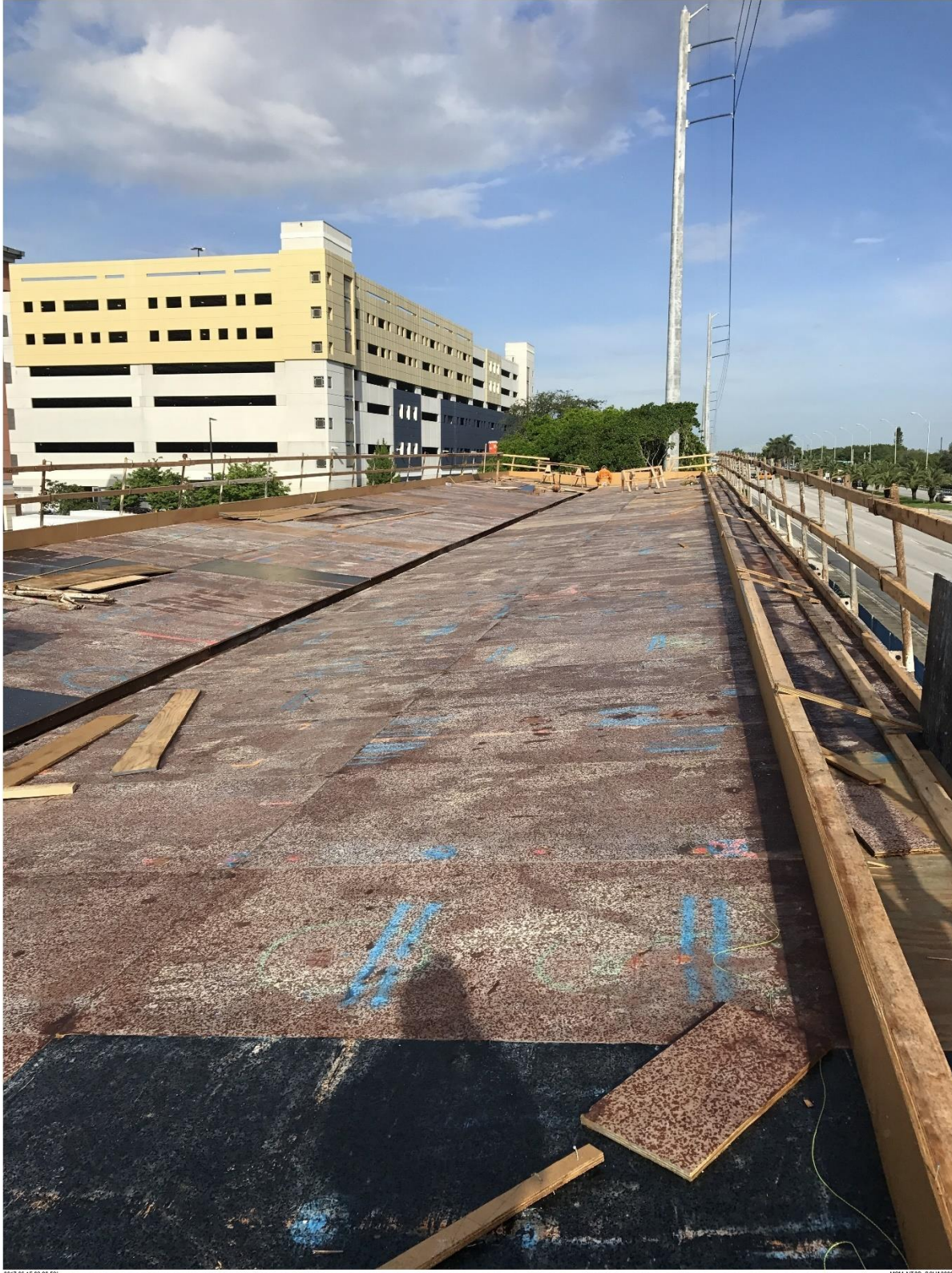
Bridge Factors Photo 4 – View of forms being set for concrete pour of main span deck on 6/15/17 at 8:39:58 a.m. (Source: Munilla Construction Management, MCM)
