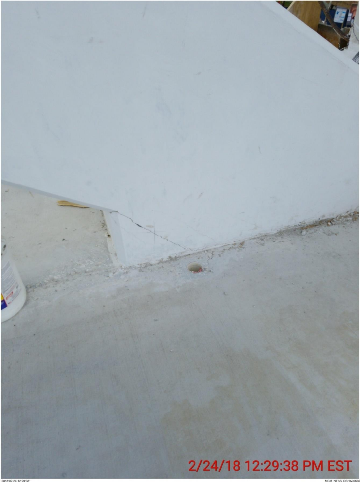
Bridge Factors Photo 38 – View of crack at the bottom of diagonal support #11 on north side looking to the south in casting yard on 2/24/18 at 12:29:38 p.m. (Source: Munilla Construction Management, MCM)
