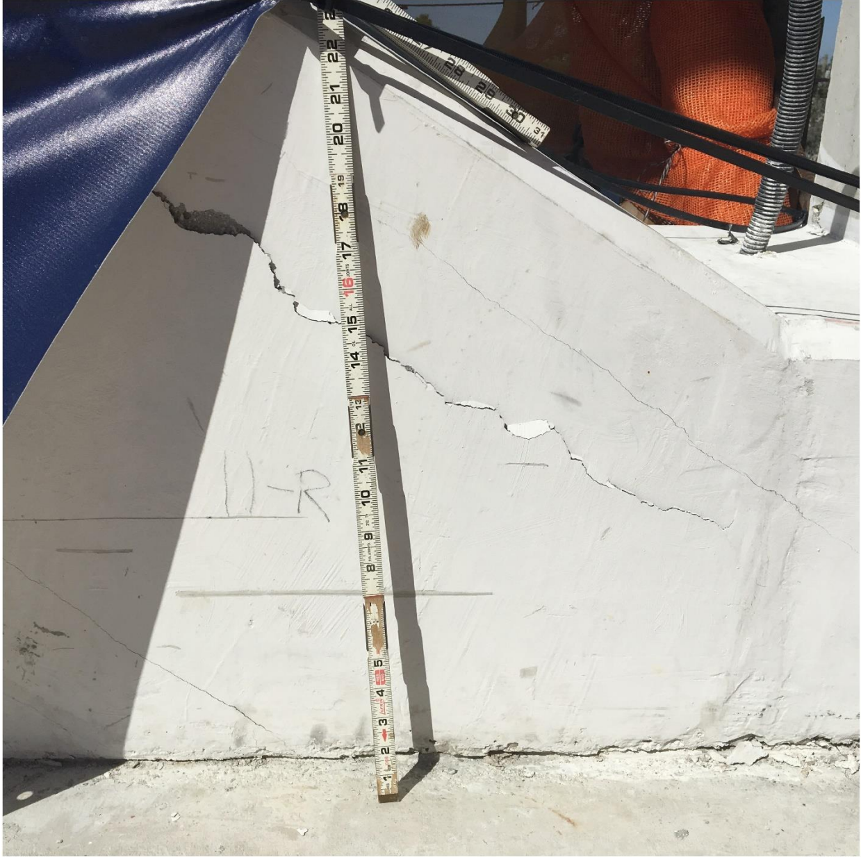
Bridge Factors Photo 78 – View of crack along bottom of diagonal support #11 on east side on 3/13/18 at 11:20:19 a.m. (Source: Munilla Construction Management, MCM)
