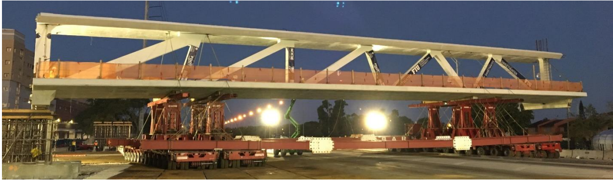
Figure 15 – Main span during move (Source: Barnhart Crane and Rigging)
