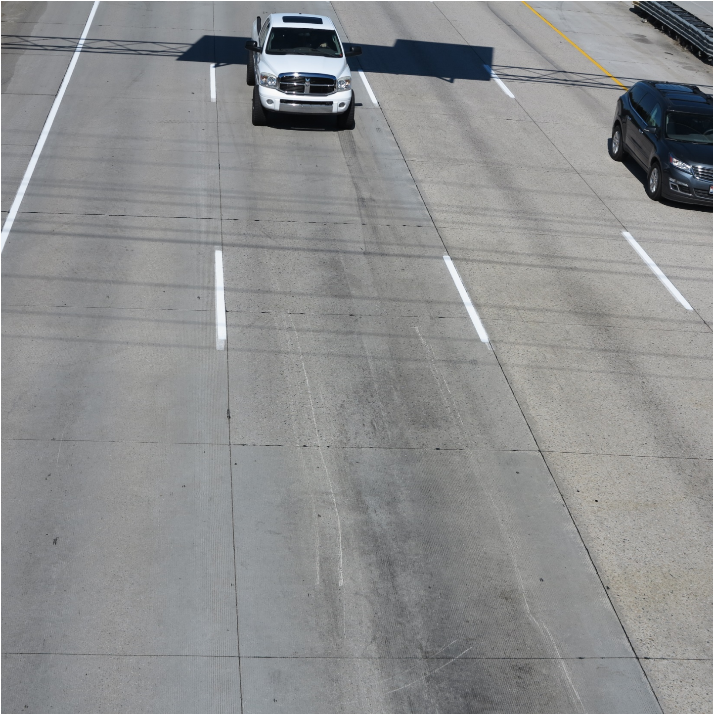
Highway Photo 10 – Additional view of tire marks and scrapes in the impact lane.
