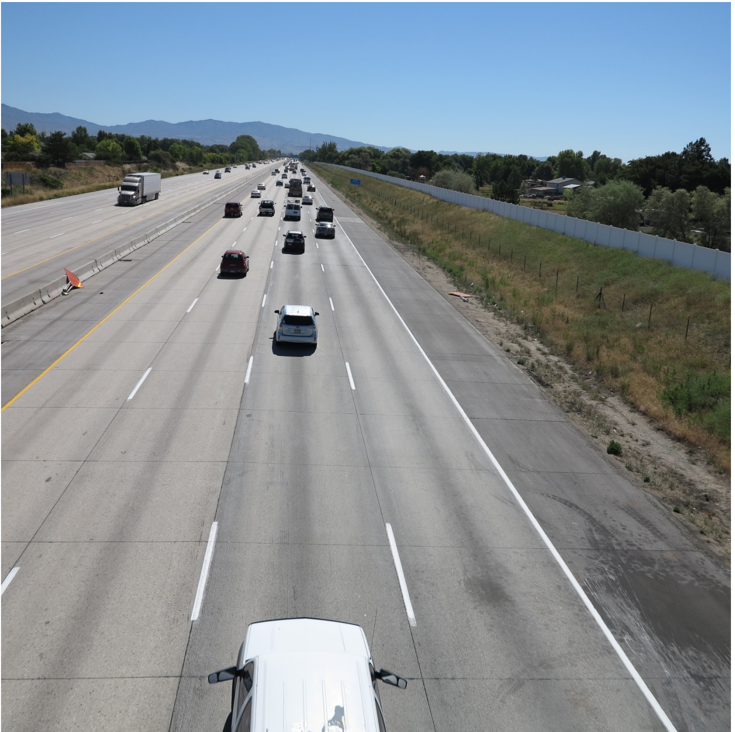
Highway Photo 13 – Eastbound view of I-84 looking east from the Cloverdale overpass. The two, “Left Three Lanes Closed” signs are visible on the shoulders of the highway.
