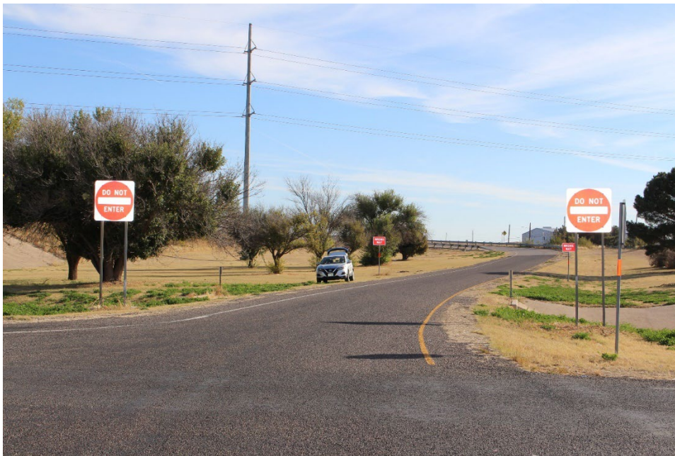
Figure 5. View of DO NOT ENTER signs followed by WRONG WAY signs on the exit ramp where the truck driver traveled to enter I-20.
