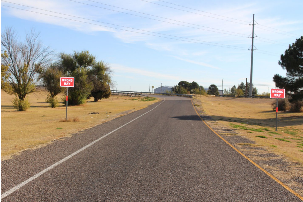
Figure 8. View of WRONG WAY signs posted 150-feet after the DO NOT ENTER signs.
