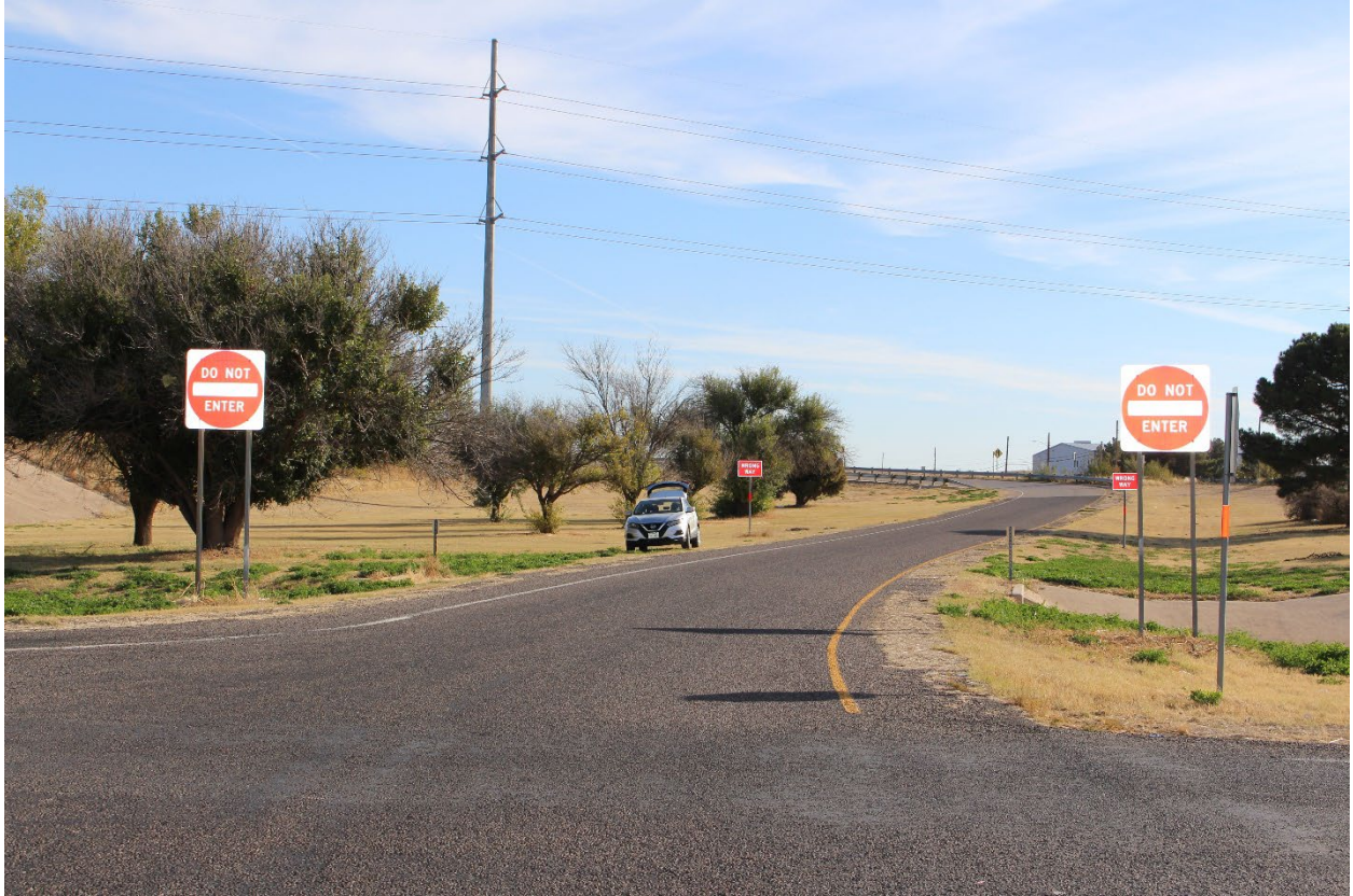
Figure 7. View of DO NOT ENTER signs followed by WRONG WAY signs on the exit ramp where the pickup driver traveled to enter I-20.
