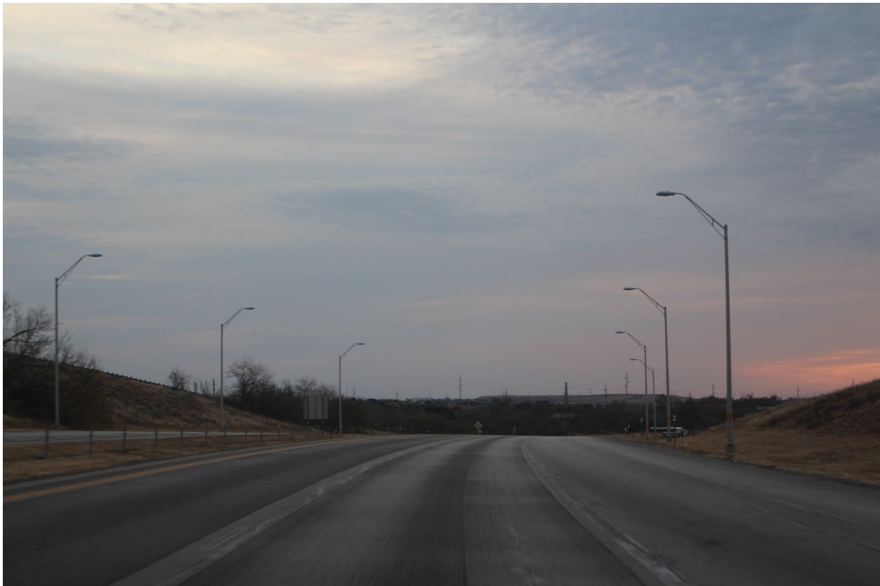
Figure 4. View of eastbound I-20 showing the horizontal and crest vertical curve on the approach to the crash location.
