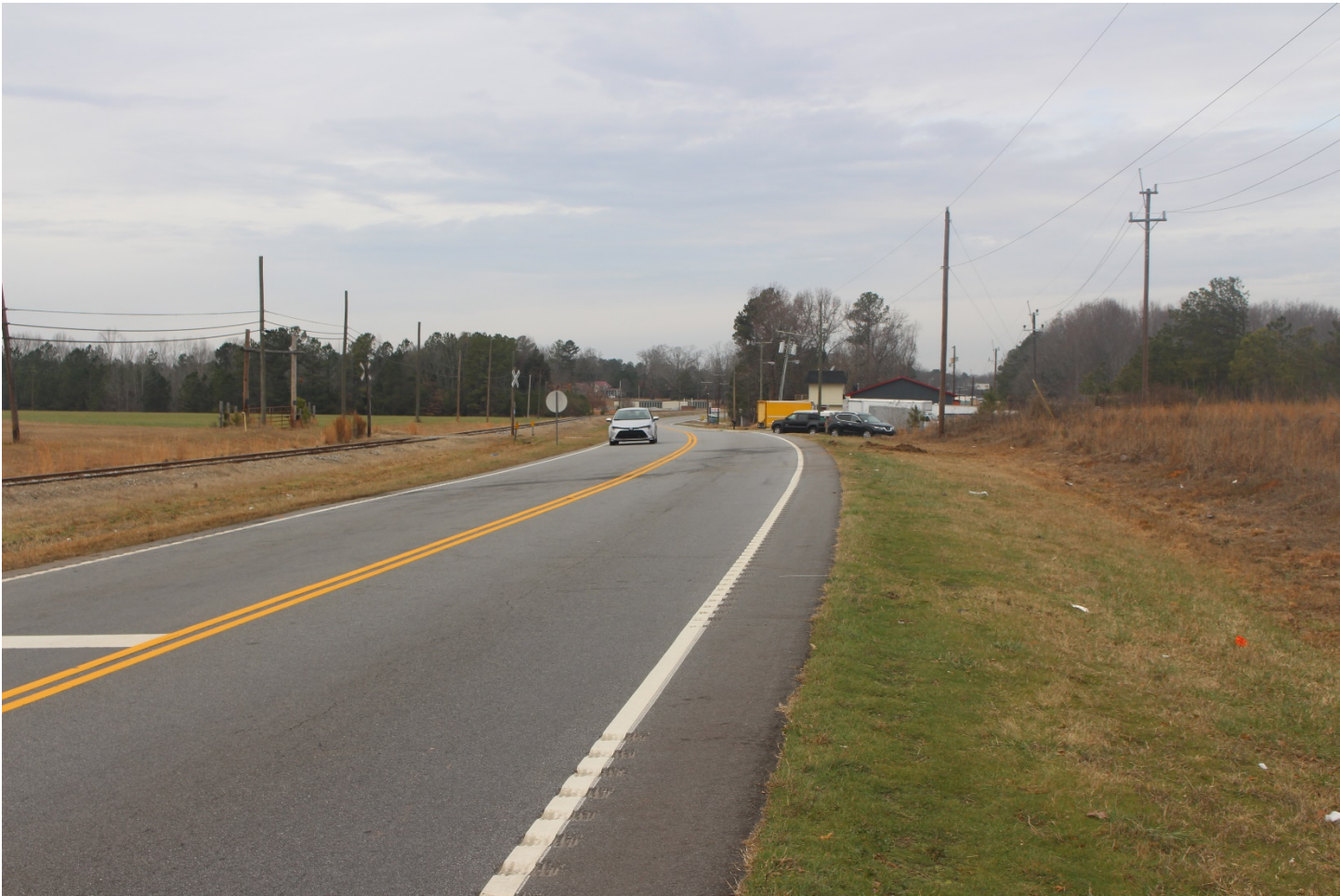
Highway Photo 8 – Closer view of curve alignment from the westbound lane.
