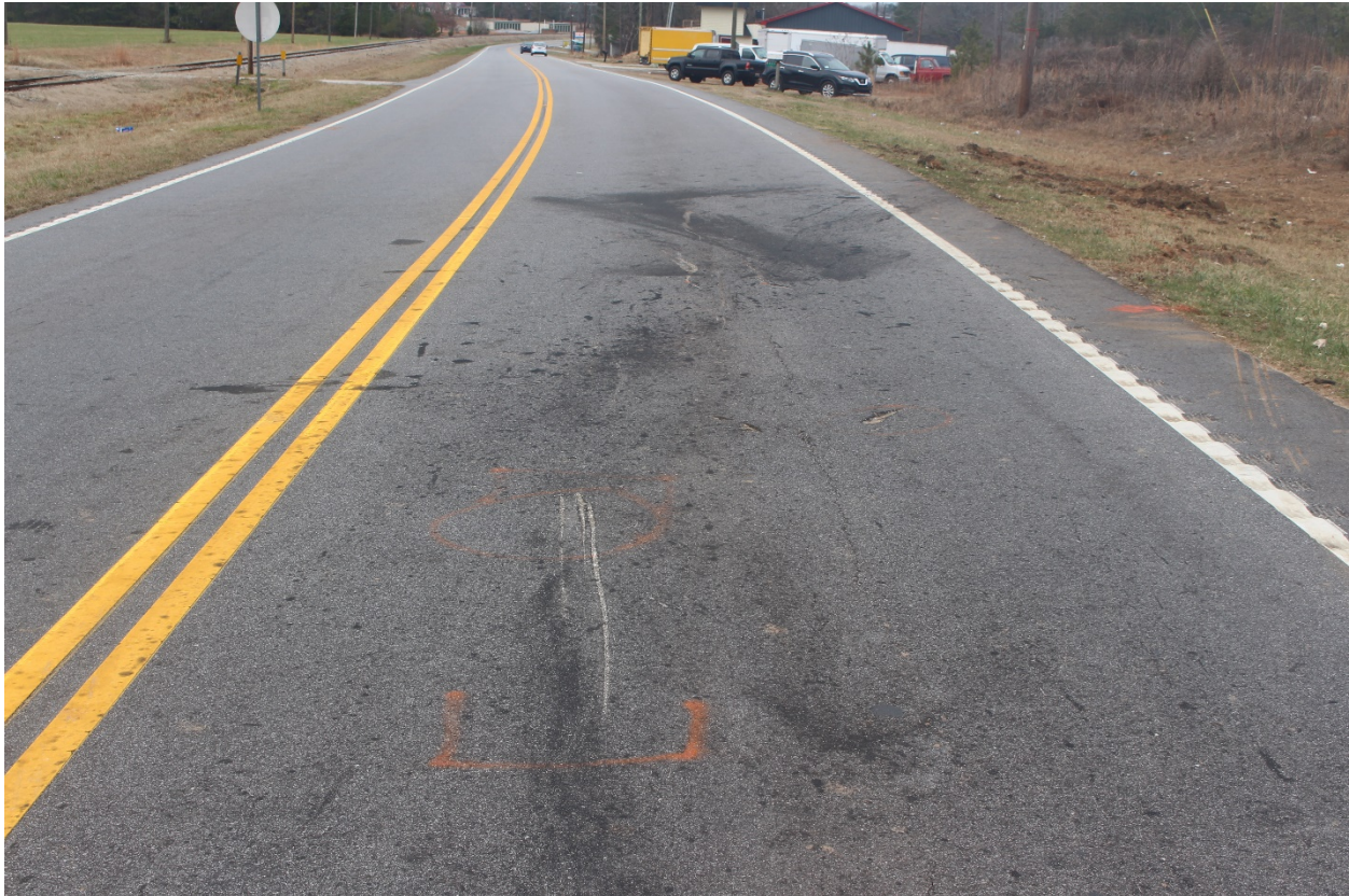
Figure 5. View of westbound US-76, showing Scrubs in bus's travel lane.
