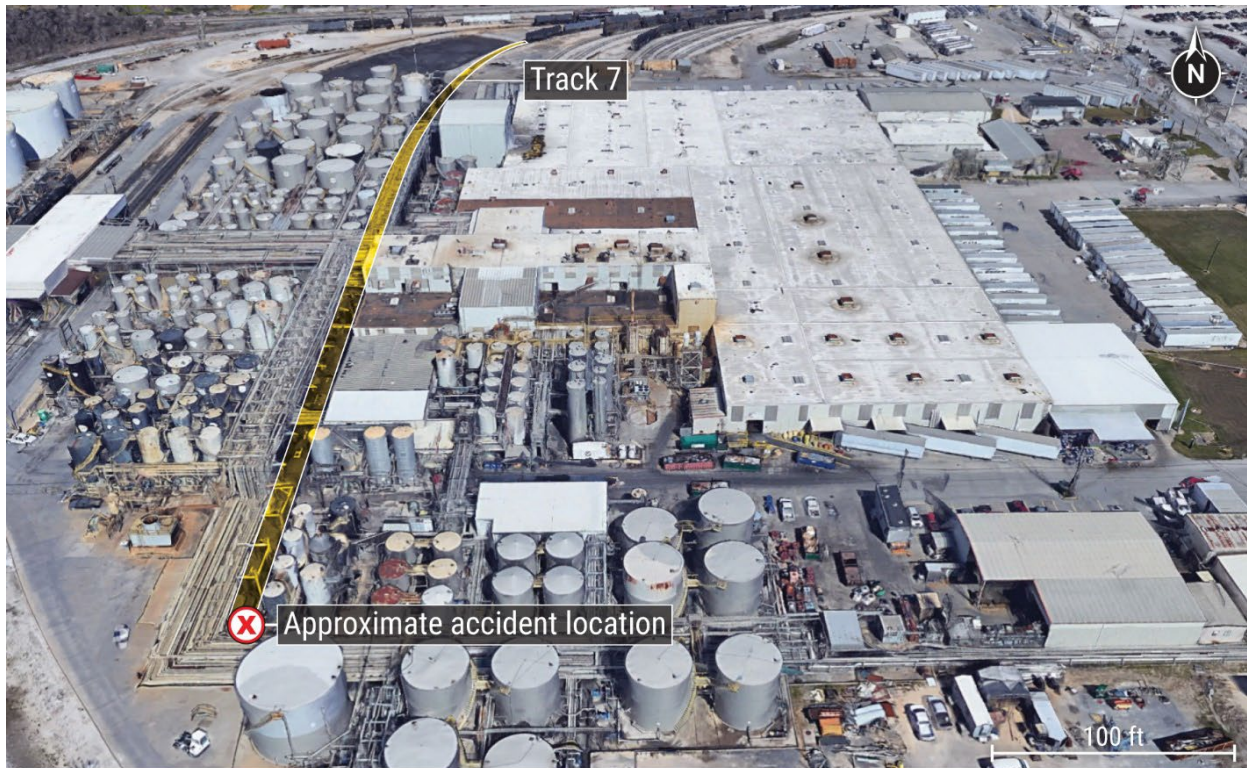
Figure. Overhead image of the accident location at the ExxonMobil refinery plant. (Source: Google Earth Pro.)
