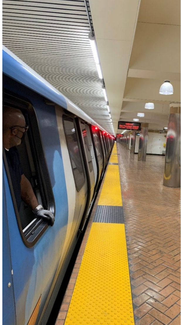
Figure 3. Powell St. Station platform after completion of lighting improvements.
