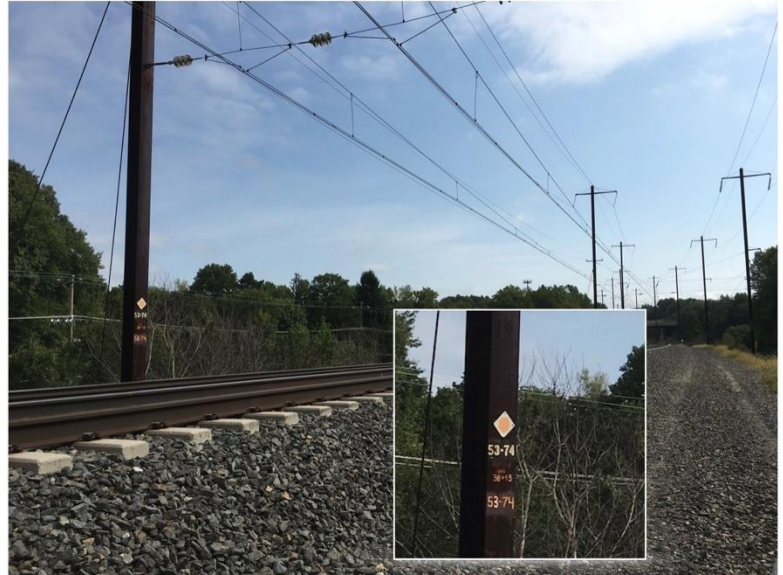
Typical decal or placard at MP 53.74 denoting Hot Spot due to limited visibility Curves 344-345 on Amtrak's Mid-Atlantic Division
