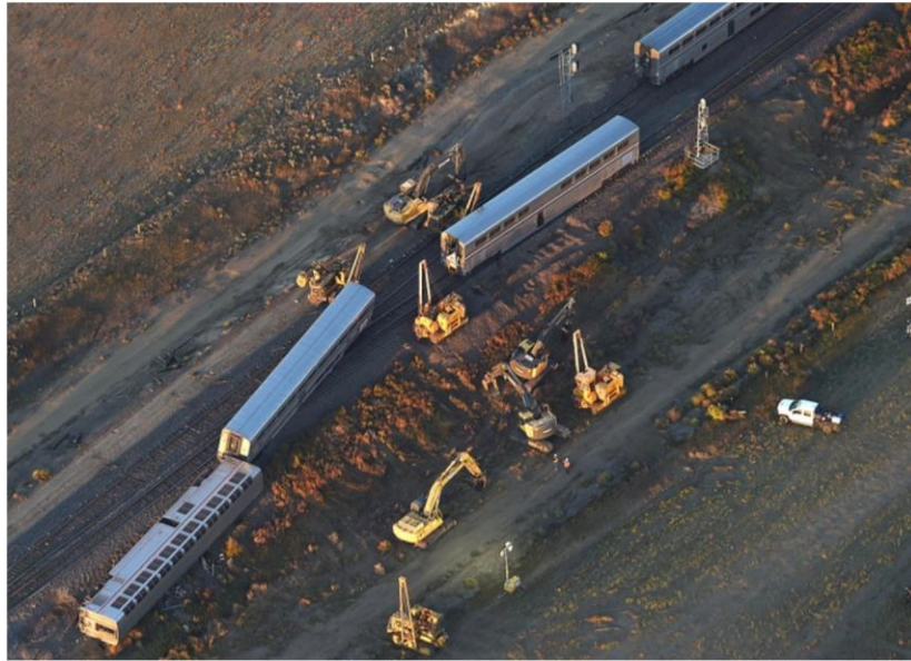
Figure 1 – Aerial photo of derailment ( Photo courtesy of Fox 4 – WDAF TV )
