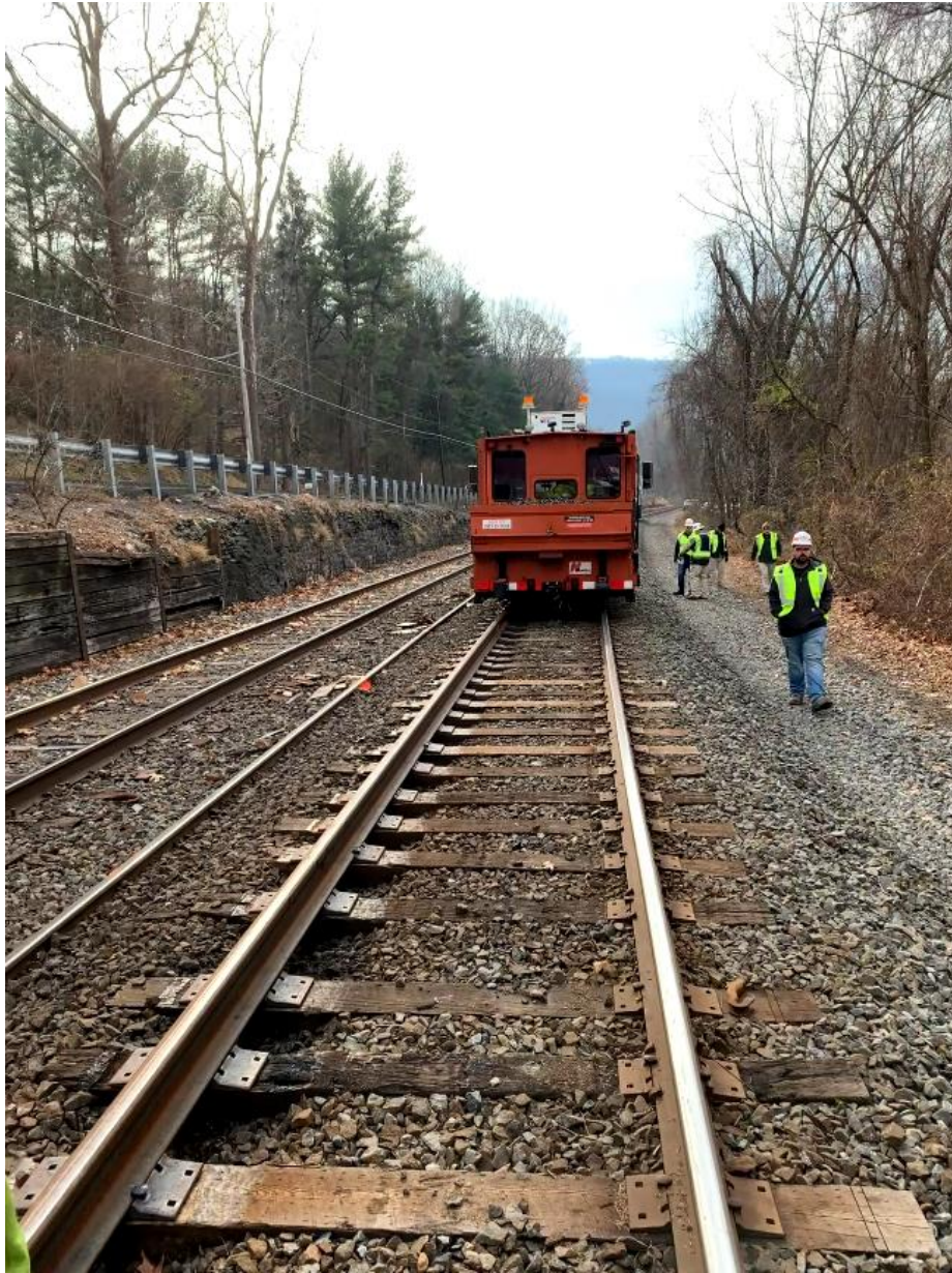
Figure 1: Rear of Spiker No. 2, viewed from the north.
