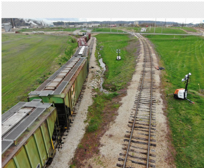
Figure 1 – Photo of accident site (Photo courtesy of NTSB)
