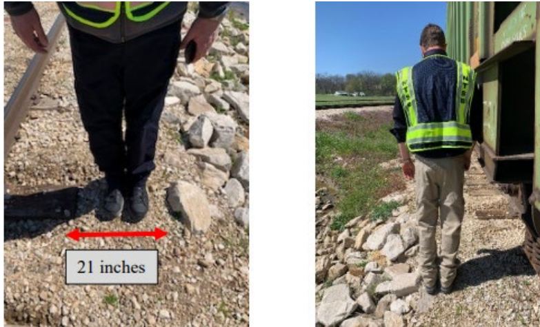
Figure 5 – Photos showing walking condition at the Dyno Nobel facility. The photo on the left shows the width of the walking space between the edge of the railroad ties and the adjacent rocks where the slide marks in the ballast were found. The photo on the right shows the walking space for an average sized person. (Courtesy of NTSB)
