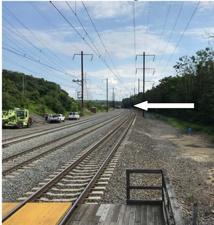
View looking North from Bowie State Platform. Arrow reflecting approximate accident location. No. 1 track is on the right side.
