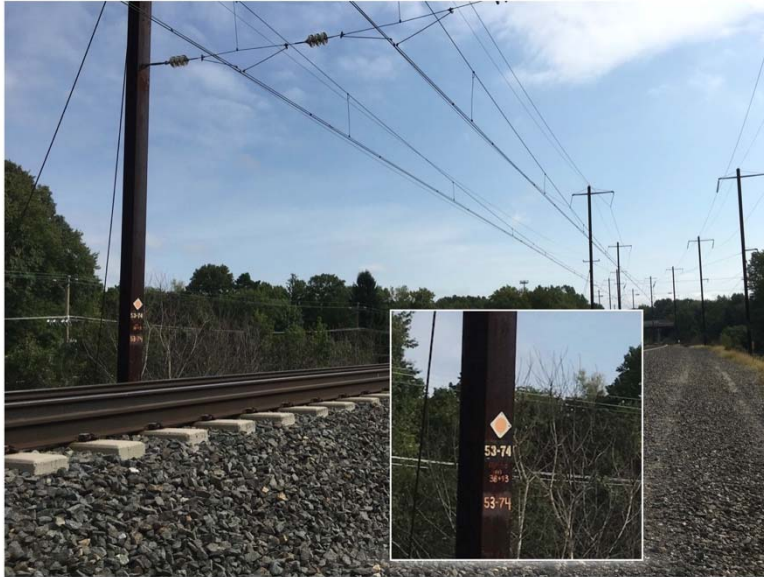
Typical decal or placard at MP 53.74 denoting Hot Spot due to limited visibility Curves 344-345 on Amtrak's Mid-Atlantic Division
