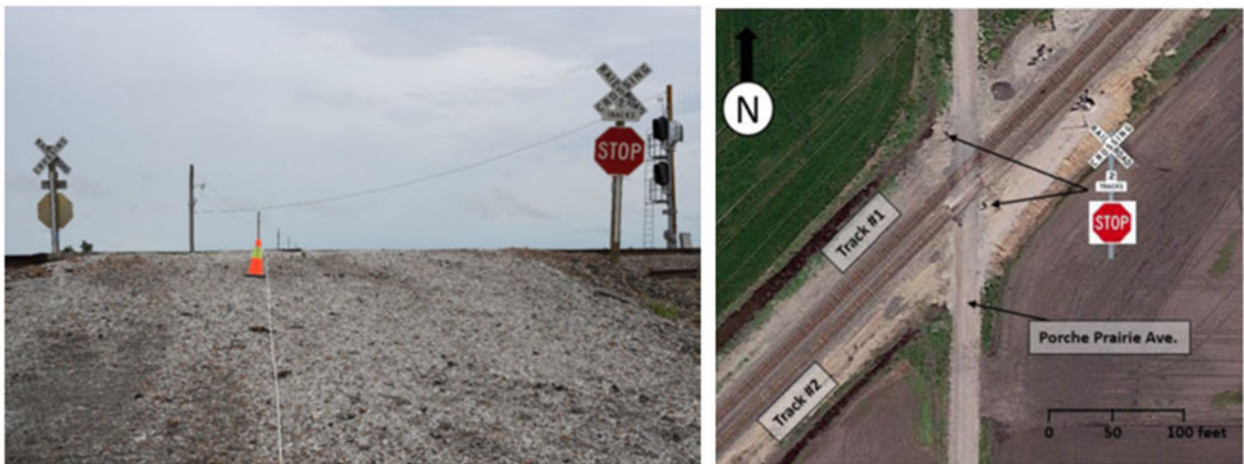
Figure 4- View of stop sign, crossbucks, and grade at Porsche Prairie crossing (Photos courtesy of Missouri Highway Patrol and NTSB Highway Factual report)
