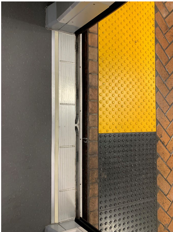
Figure 6: Platform edge gap at Powell St. Station
