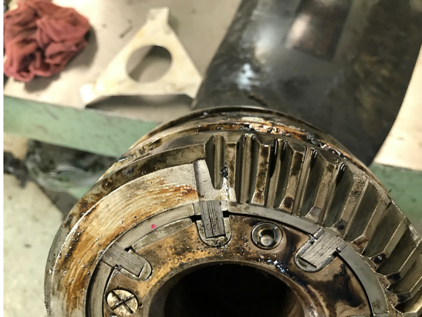
Photo No. 210: Close up of No. 3 blade butt showing the gear segment was intact and the screws in place.
