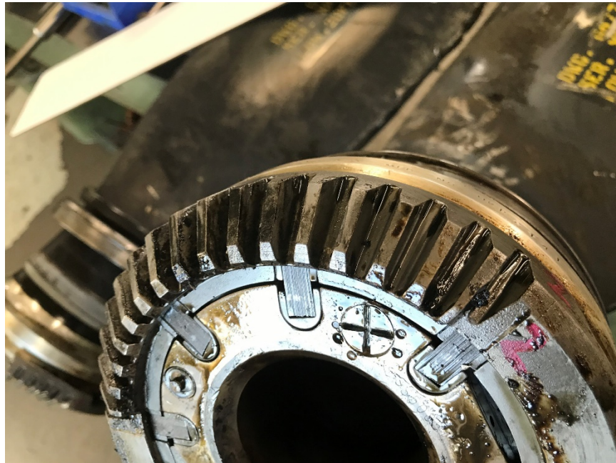
Photo No. 208: Close up of No. 2 blade butt showing the gear segment was intact and the screws in place.
