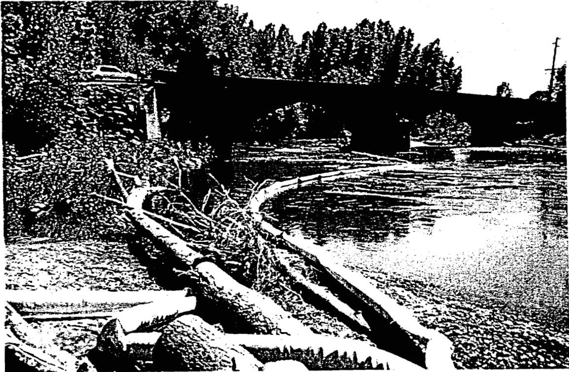
Initial boom deployment at Mounts Road.
