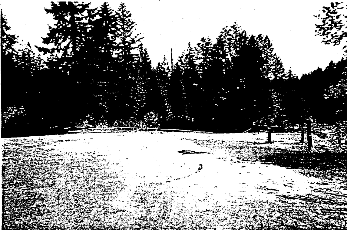
Recondo 2 does have plenty of room for equipment staging.
