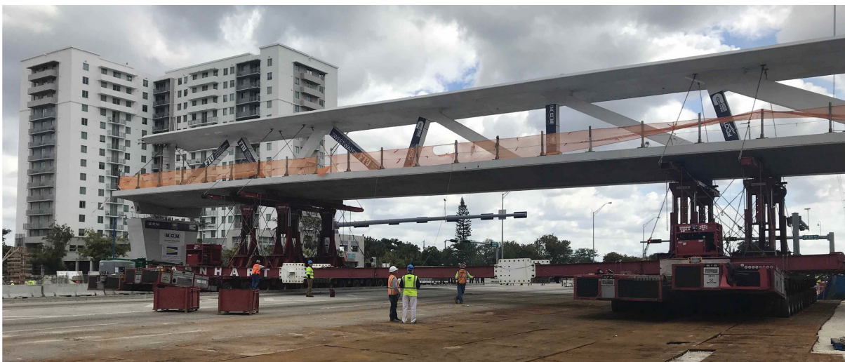
Figure 15. Photograph showing SPMT transport of the bridge.
