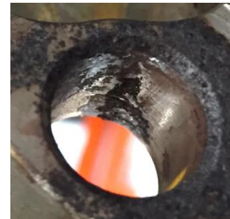
HPC case S5 Borehole
