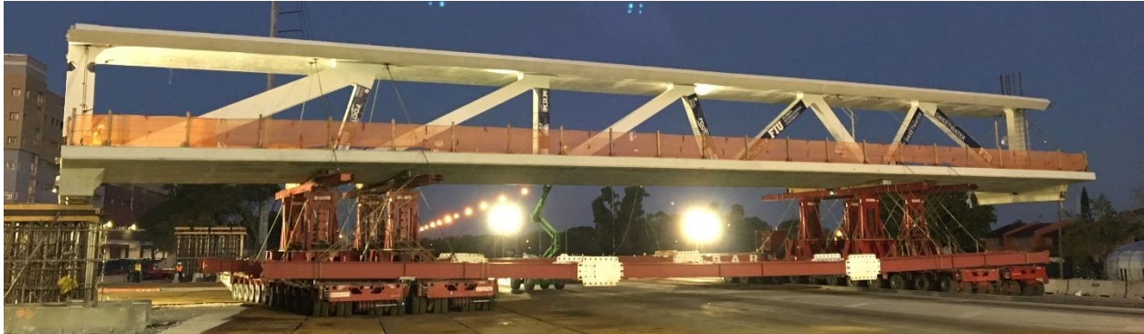
Figure 2 - Main Span During Move
