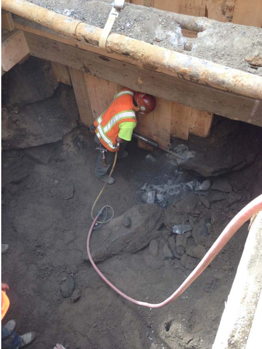
Figure 2: Excavation for the sewer connection at 1642 Park Avenue continued to show boulders in backfill materials being split with drill. Sources NYCDEP.
