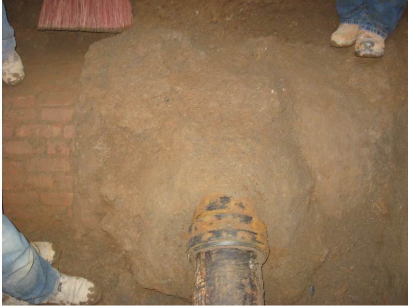
Figure 5: Close top view of direct connection of 1642 Park Avenue Sewer lateral into the combined Sewer Main without “a riser”. Source: NYCDEP
