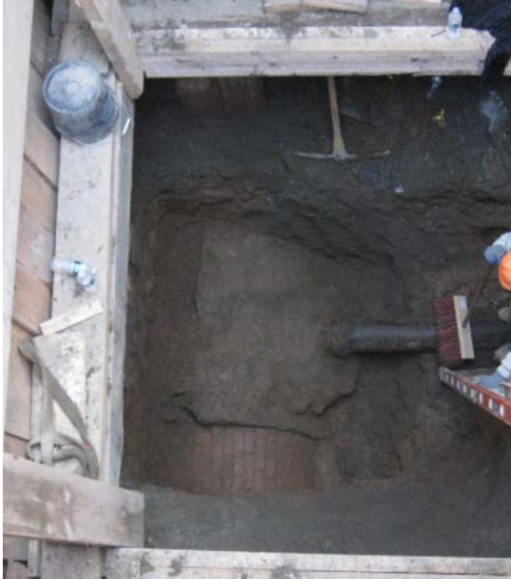
Figure 3: Direct Connection of 1642 Park Avenue lateral into the combined Sewer Main without “a riser”. Source: NYCDEP
