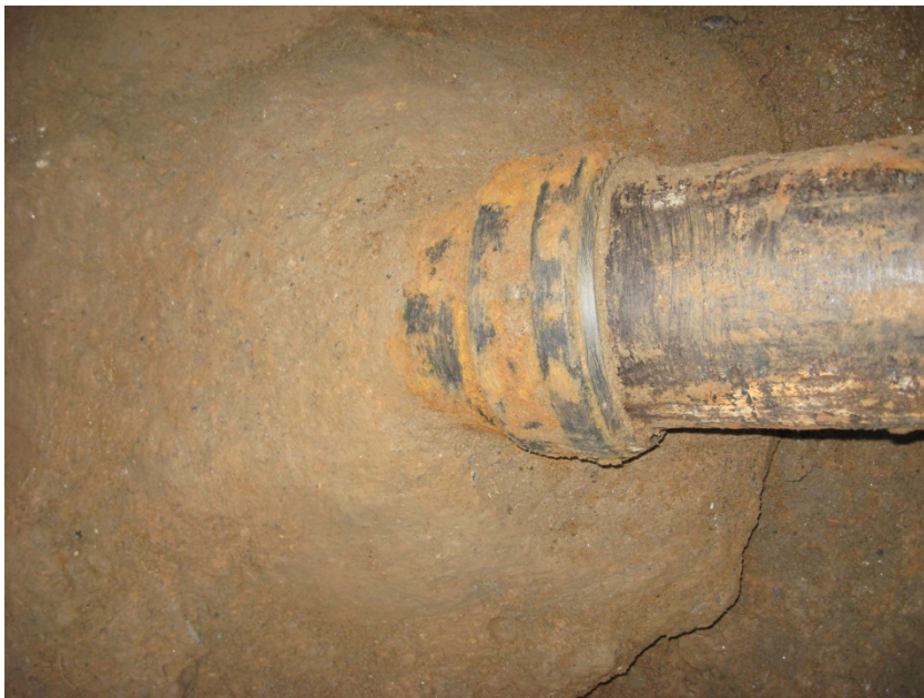
Figure 4: Close north side view of direct connection of 1642 Park Avenue Sewer lateral into the combined Sewer Main without “a riser”. Source: NYCDEP
