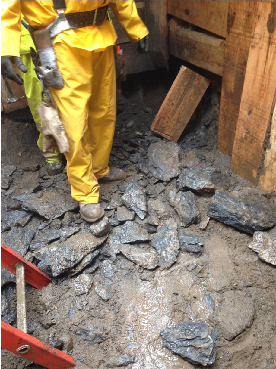
Figure 1: Excavation for the sewer connection at 1642 Park Avenue revealed presence of boulders in the backfill materials. Source: NYCDEP
