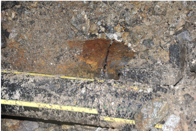
Figure 6: Excavation shows both 12-inch water main break location and 8-inch HDPE during emergency response excavation. Source: FDNY
