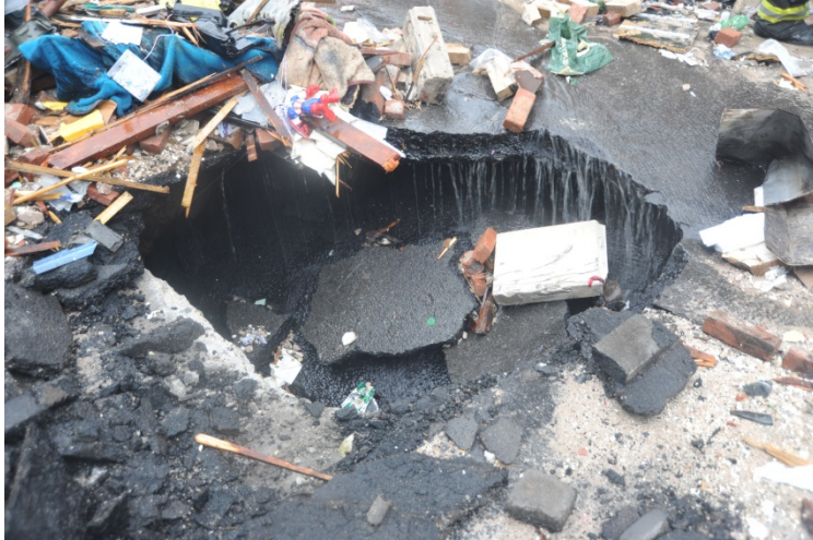
Figure 1: Sink-hole observed at the location of the 12-inch water main break, 8-inch HDPE gas main opposite 1642 Park Avenue during emergency response excavation. Source: FDNY
