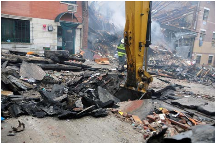
Figure 4: Excavator bucket clearing pieces of roadway pavement (asphalt and concrete) from cavity at 8-inch HDPE gas main, 2-inch HDPE gas service tee to 1642 Park Avenue and 12-inch cast iron water main location during emergency response excavation. Source: Con Edison
