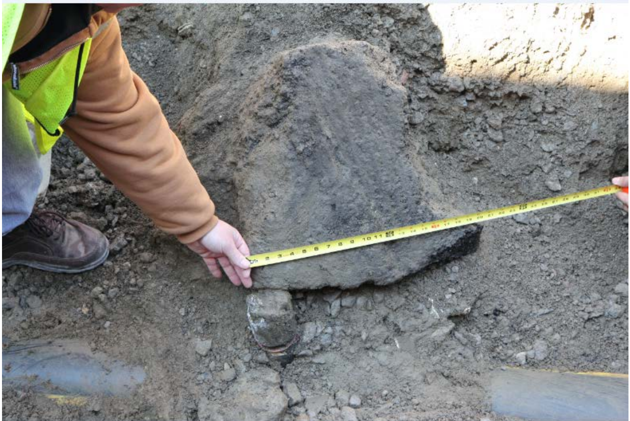
Figure 8: Re-excavation at 1642 Park Avenue show asphalt piece on top of service saddle tee cap that measured about 14-20 inches wide during field investigation. Source: NYPSC
