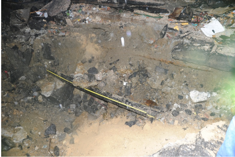
Figure 5: Excavation shows both 12-inch water main break location and 8-inch HDPE going south to 1642 Park Avenue Service tee about 9 feet from water main crack during emergency response excavation. Source: FDNY
