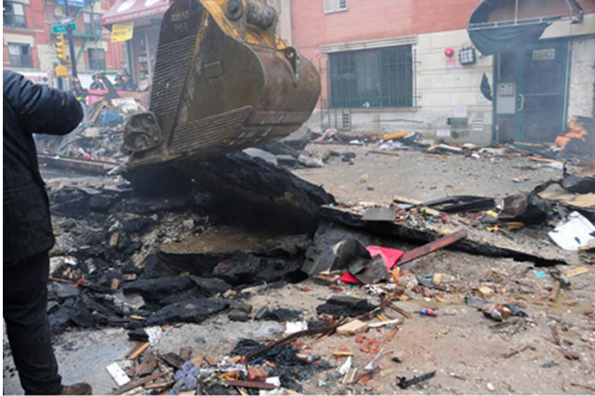
Figure 3: Excavator removing asphalt over 8-inch HDPE gas main, 2-inch HDPE gas service tee to 1642 Park Avenue and 12-inch cast iron water main during emergency response excavation. Source: Con Edison
