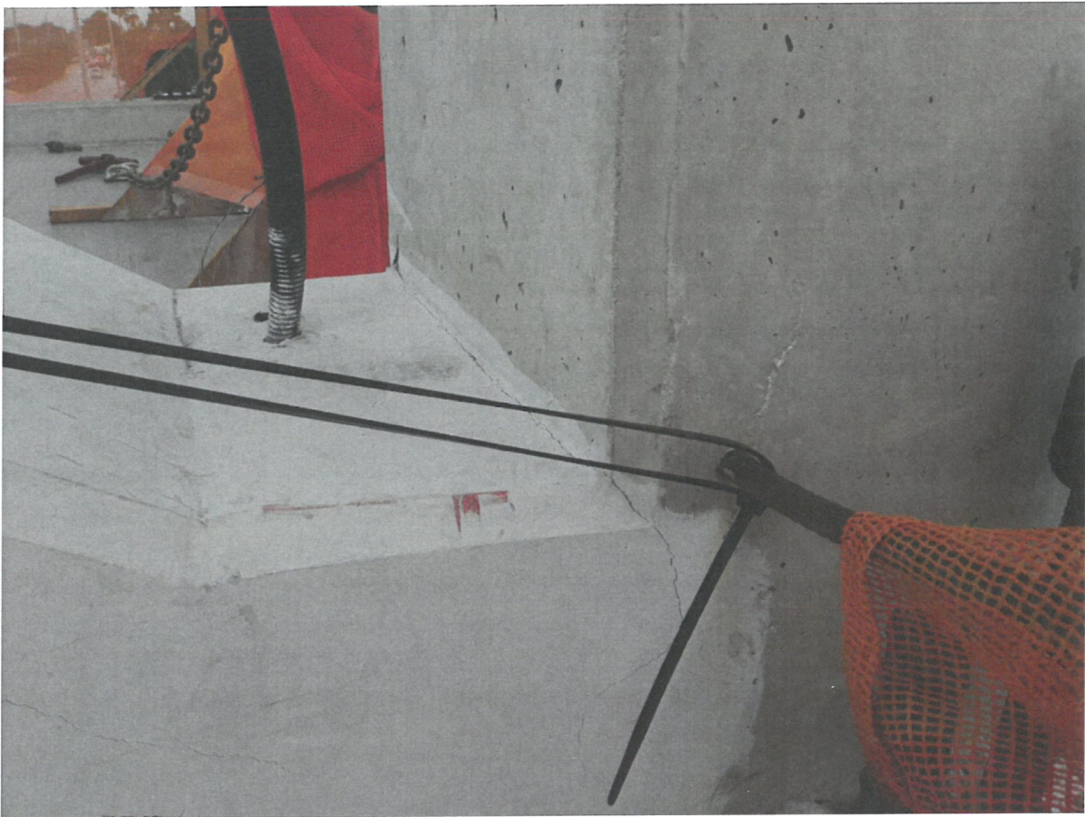
PHOTO 4: Truss 11/12 crack
