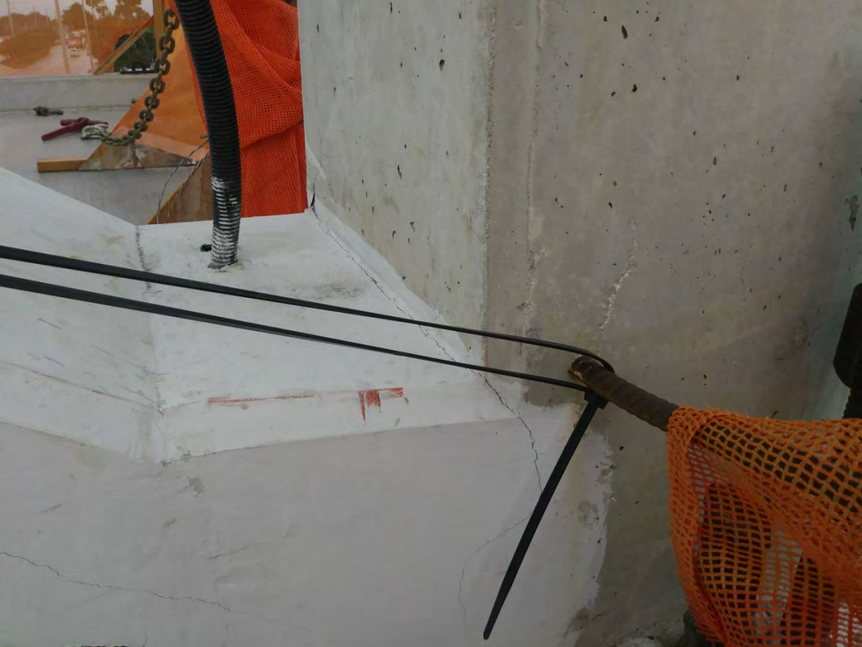
PHOTO 4: Truss 11/12 crack
