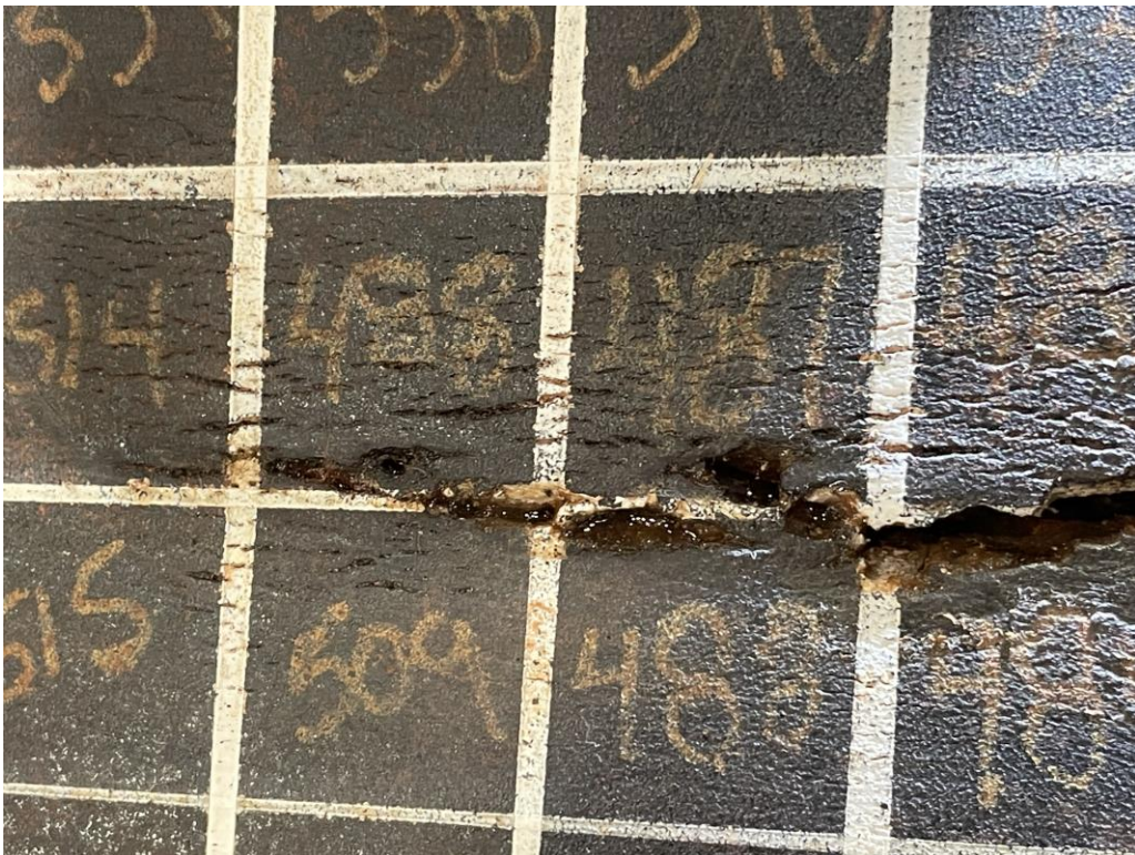
OD surface prior to MT
