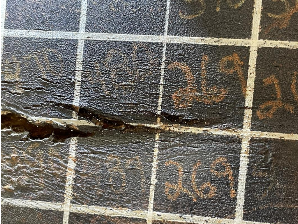
OD surface prior to MT
