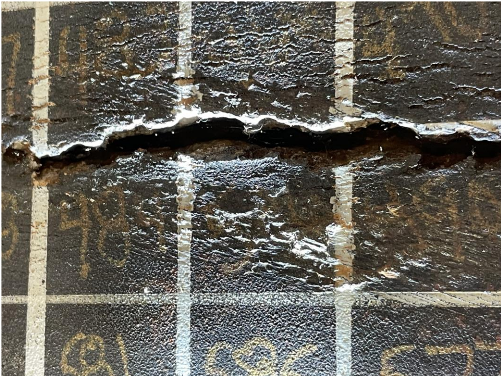
OD surface prior to MT
