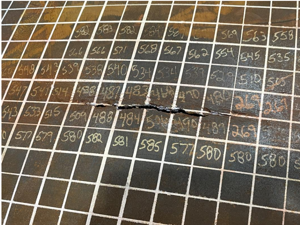
OD surface prior to MT
