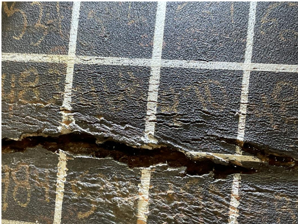
OD surface prior to MT
