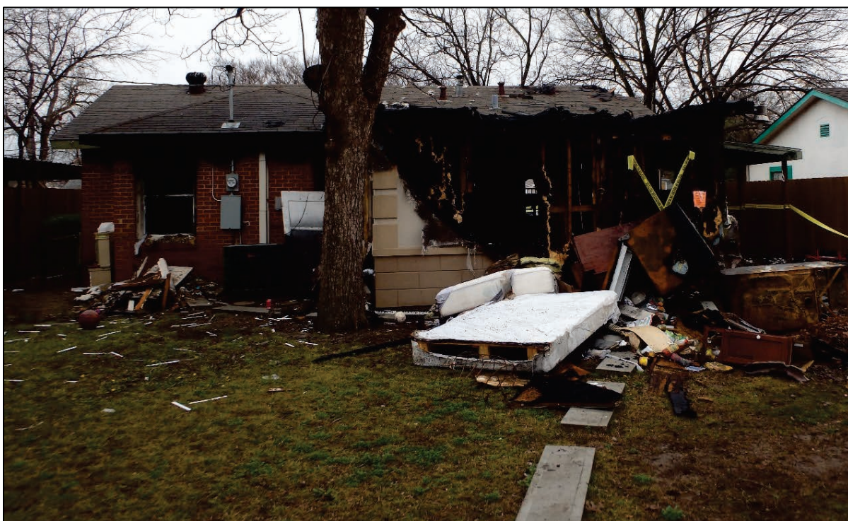
Figure 17. Back of 3515 Durango Drive. Photo by DFR.
