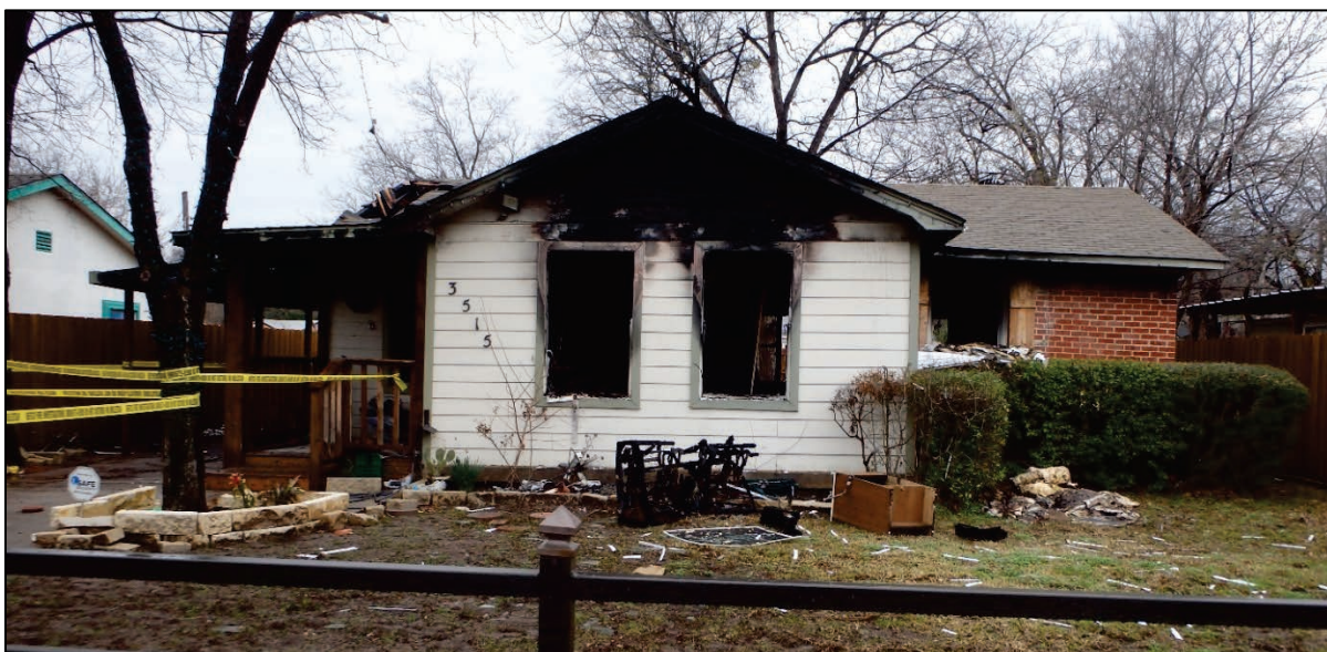
Figure 16. Front of 3515 Durango Drive. Photo by DFR.
