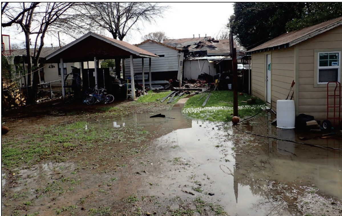
Figure 15. Photo of 3527 Durango Drive Taken by Atmos Energy on 2/24/2018. Image is taken from rear facing the back of the house. Standing water is shown in backyard.
